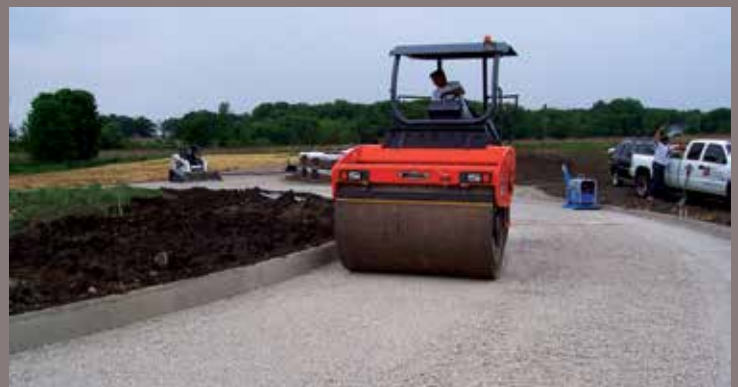
(Above) A worker is using a large, vibratory smooth drum roller to compact the open-graded aggregate base on this roadway. The equipment is appropriately sized for the job.
