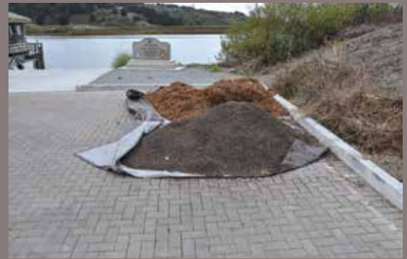
Here, landscaping materials, such as topsoil and wood chips, are piled on tarps placed on the surface of the permeable pavement. This approach is an example of good protection of the PICP during construction.
