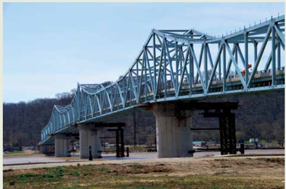
Milton-Madison Bridge Project
