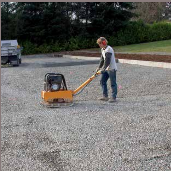
(Left) This construction worker is compacting an open-graded aggregate base in a parking lot using a plate compactor that is too small for the size of the project. A roller compactor would be more efficient.
