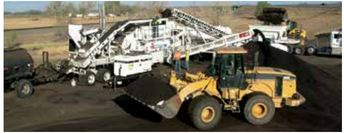
A construction crew uses in-place recycling equipment, shown here, beside a stockpile of reclaimed asphalt pavement.
