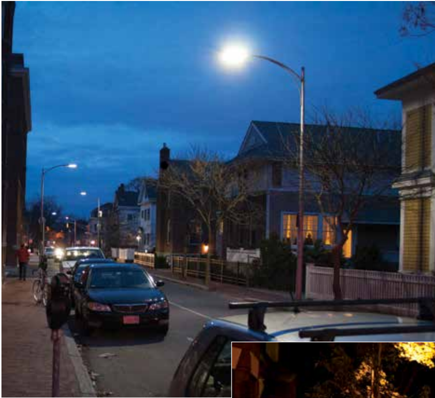
The city of Cambridge, MA, installed new LED fixtures operated by an adaptive control system along this residential street. The new luminaires (left) make colors look brighter and more faithful to the natural color, improving visibility even when the amount of light is less than with the old lights (below). Photos: Paul Lutkevich, Parsons Brinckerhoff.
