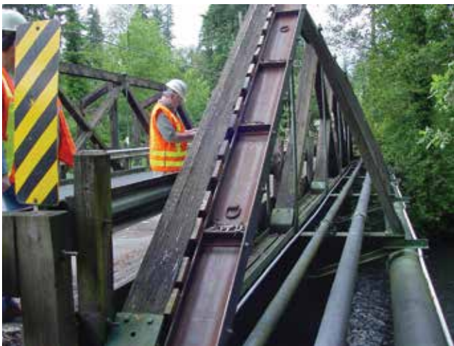
FHWA has started collecting additional data to better monitor the condition of bridges, such as this one being checked by an inspection team.
