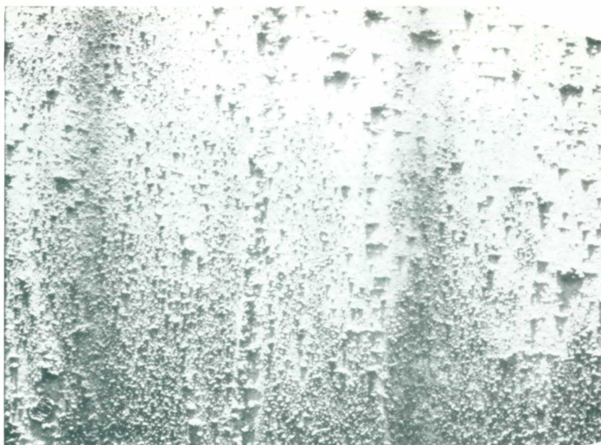
a. HULL CONDITION PRIOR TO CLEANING
