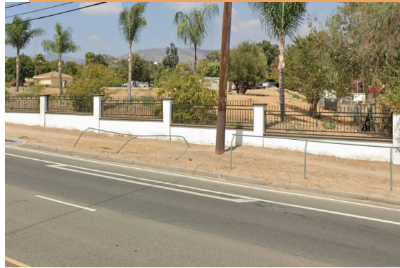
Figure 5: Bent Metal Bars on Bridle Path along Foothill Blvd.
