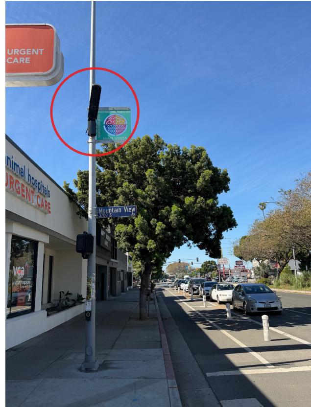
Above: LADOT's Permanent Bike Counter attached to a light post on the South side of Venice Boulevard.
