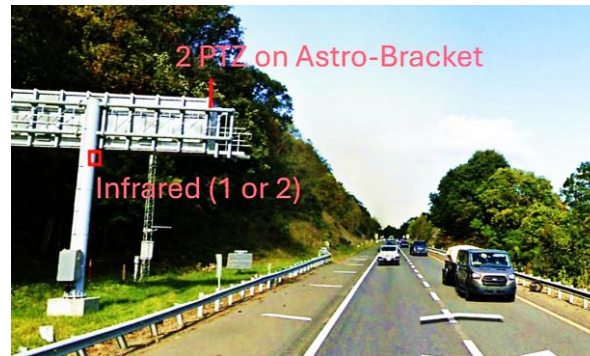
Figure 3. Camera and Infrared Illumination Mounting Location. PTZ = pan-tilt-zoom camera.
