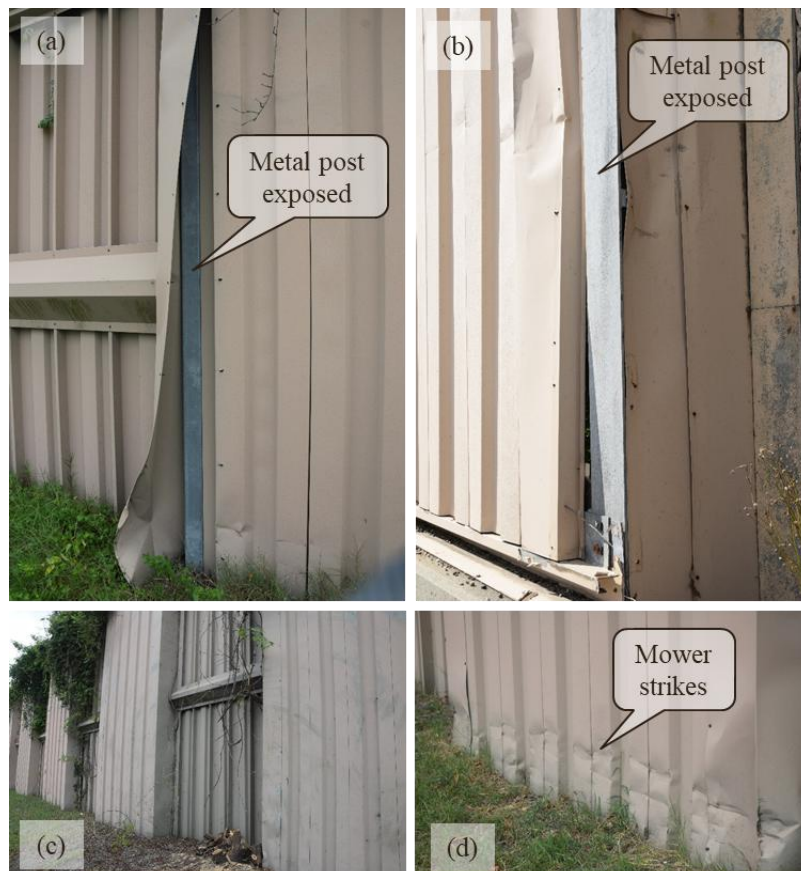
Figure 6. Additional Photos of the Condition of Noise Barriers Constructed with Metal Panels Oriented Vertically: (a) Impact Damage Leaving Metal Post Exposed on Ground-Mounted Barrier; (b) Impact Damage Leaving Metal Post Exposed on Bridge-Mounted Barrier; (c) Vegetation Growth; (d) Mower Impact Strikes on Ground-Mounted Barrier
