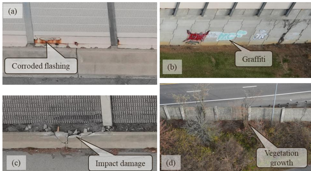
Figure 20. Screenshots of Colorized Mesh Model of Noise Barriers at Christiansburg Site: (a) Corroded Flashing at Base of PVC Noise Barrier; (b) Graffiti on Retaining Wall Below PVC Noise Barrier; (c) Impact Damage on Concrete Noise Barrier and Concrete Barrier; (d) Vegetation Growth Behind Concrete Noise Barrier. Photos were taken with a 61 megapixel camera at either 180 or 250 feet above ground level. PVC = polyvinyl chloride.
