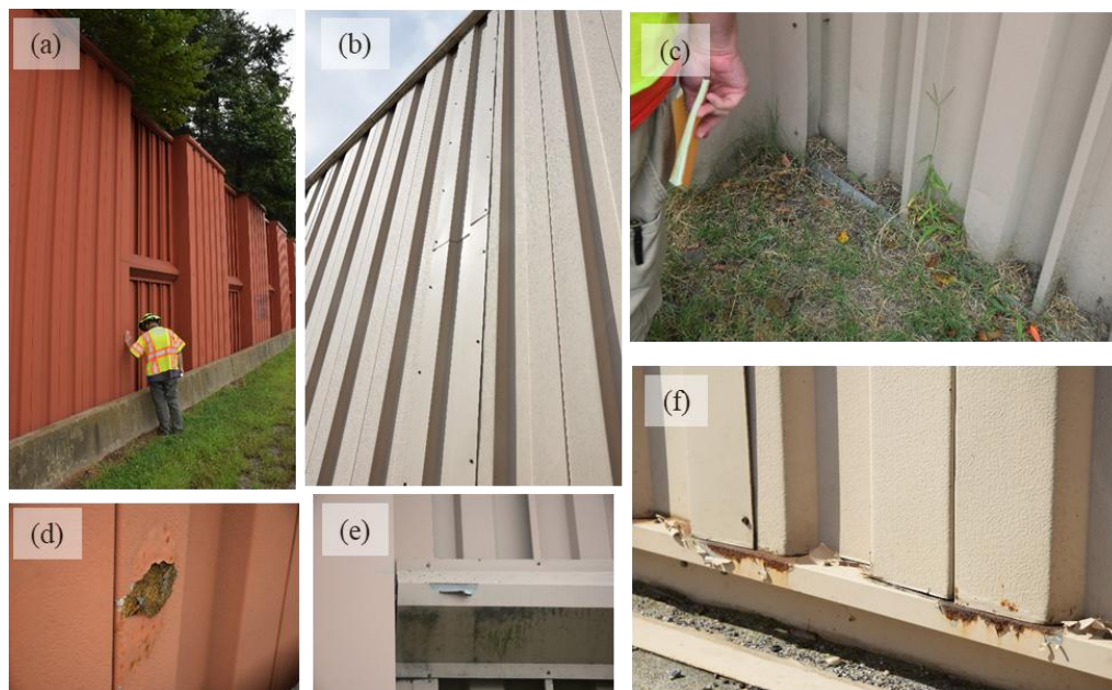
Figure 5. Photos of the Condition of Noise Barriers Constructed with Metal Panels Oriented Vertically: (a) Overall Condition of Ground-Mounted Barriers; (b) Overall Condition of Bridge-Mounted Barriers; (c) Susceptibility to Corrosion if Ponding Were to Occur; (d) Minor Section Loss at Intermittent Locations; (e) Minor Coating Failure at Intermittent Locations; (f) Corrosion Damage at Base and Flashing of Bridge-Mounted Barriers
