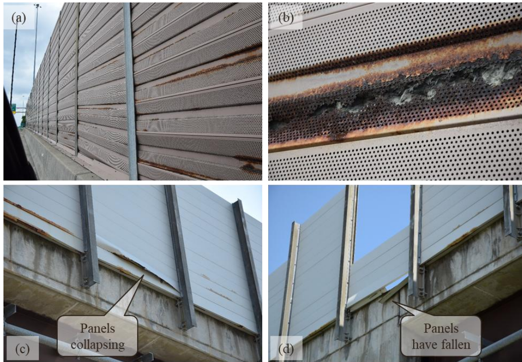
Figure 7. Photos of the Condition of Noise Barriers Constructed with Metal Panels Oriented Horizontally with Perforations: (a) Overall View from Roadway Side of Corrosion Present Throughout; (b) Closeup from Roadway Side of Corrosion Damage on Front Face of Panels; (c) Panels Collapsing Viewed from the Back Side; (d) Back Side View Showing Missing Panels that Have Fallen to the Ground
