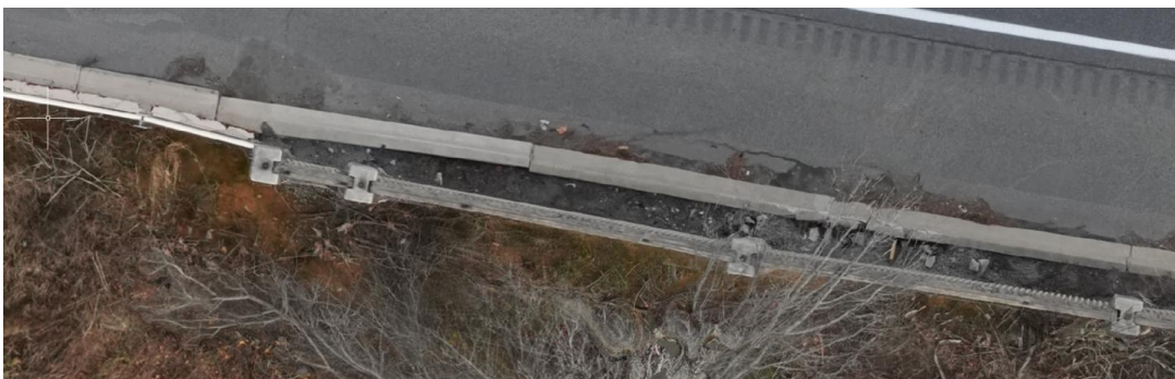
Figure 19. Orthomosaic “Top of Wall” Photo Where the Polyvinyl Chloride and Concrete Noise Barriers Join at Christiansburg Site
