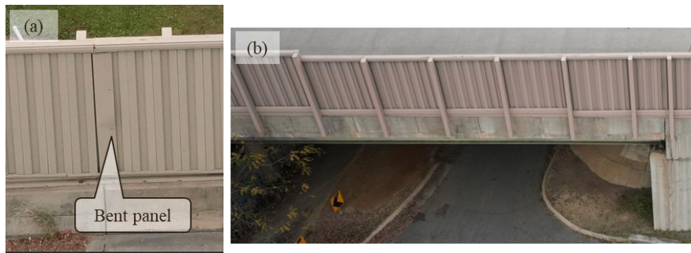
Figure 24. Screenshots from Colorized Mesh Model of Metal Noise Barrier at Fredericksburg Site: (a) Bent Panel on Front Side of Noise Barrier; (b) Back Side of Noise Barrier
