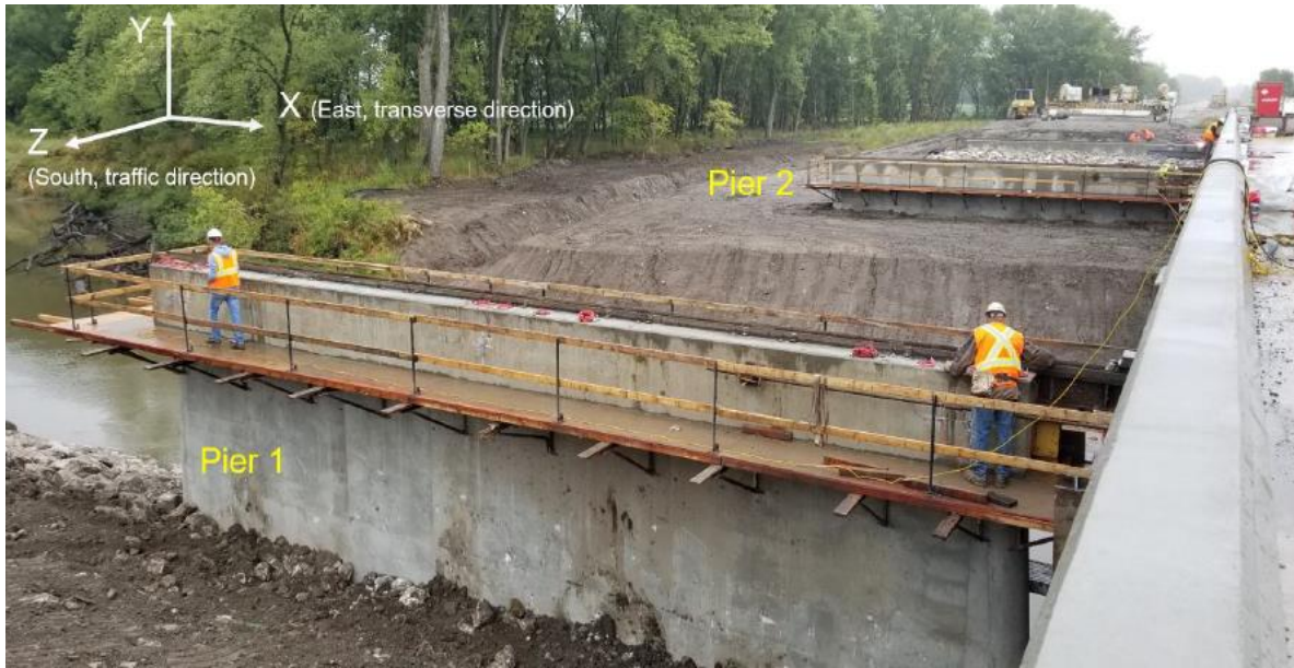
(a) Superstructure of IA 1 bridge
