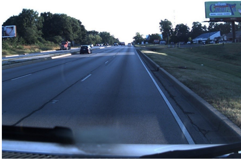
Figure 6.11 US 31 Test Section.
