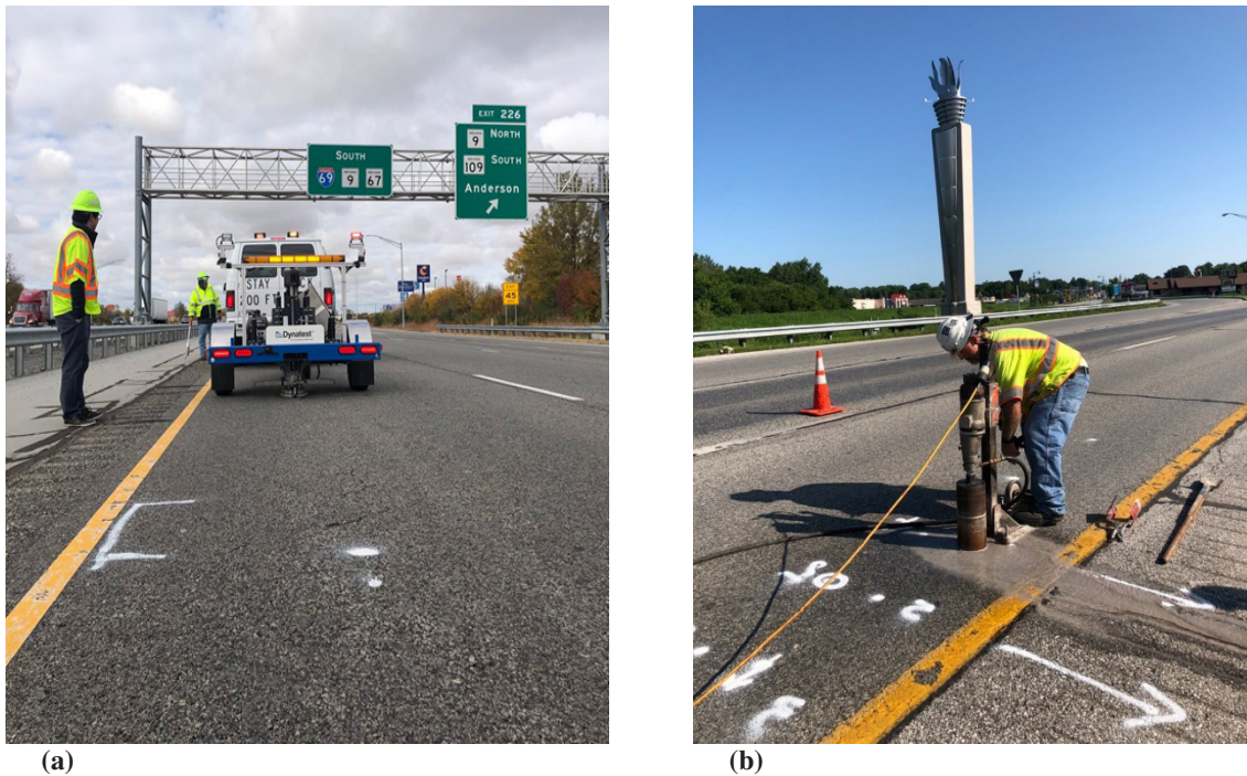
Figure 3.2 (a) FWD Testing and (b) Field-Core Sampling (I-69 Test Section).
