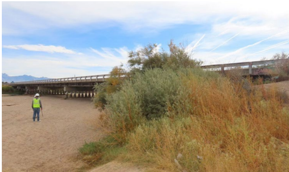
Figure 11. Profile view of the second bridge facing south (NBI number: 06255)
