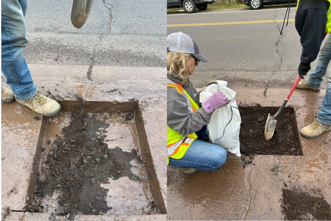
Figure 4.30: Base materials collection from the project site
