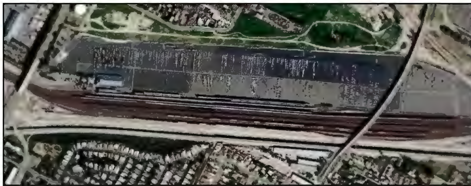
Exhibit 66: BNSF Auto Facility, San Bernardino
