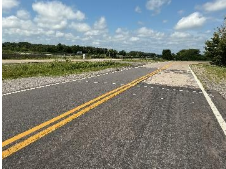
Figure 81. Settlement section of HMA next to PCC in MnROAD.
