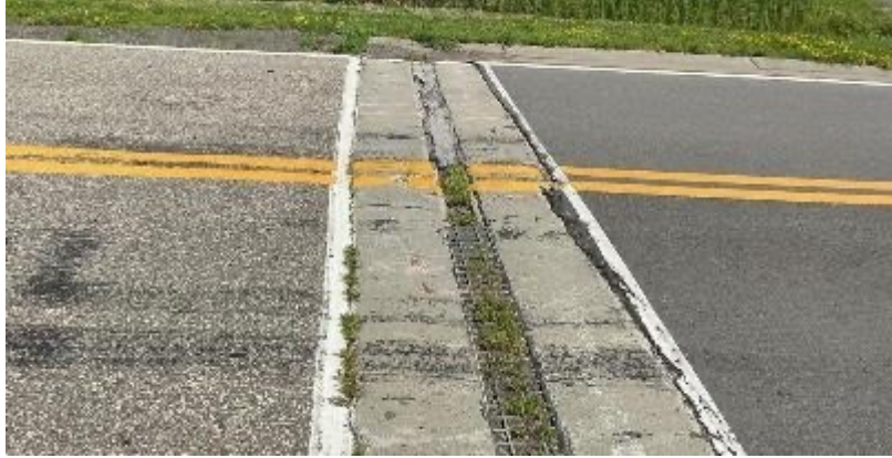
Figure 84. PCC Drain Between HMA Cells.
