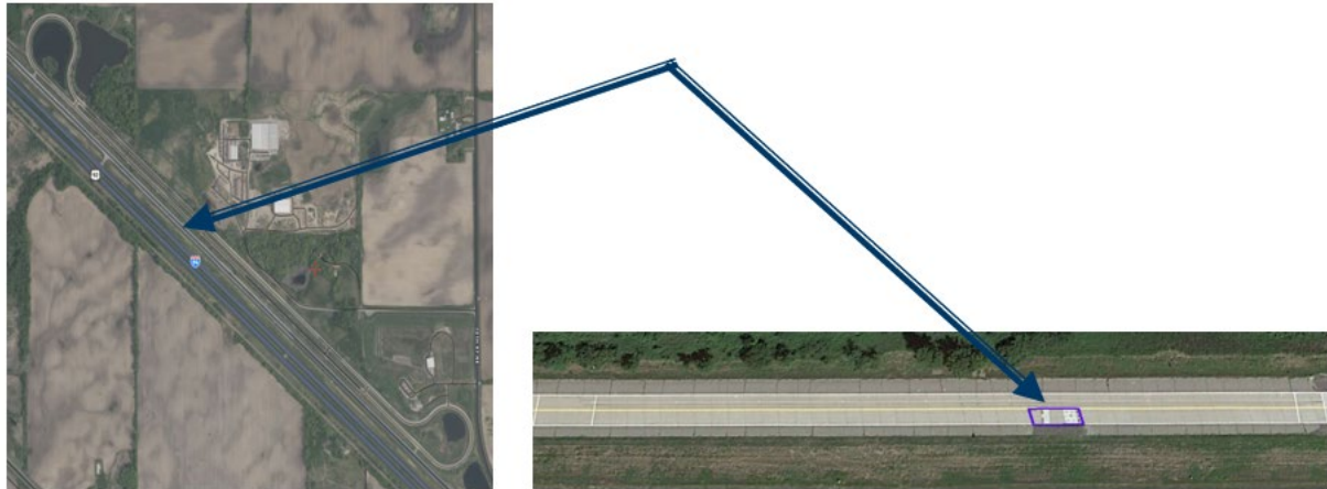
Figure 3.6 Aerial view of the low volume road and inset: Cell 2437 in perspective
