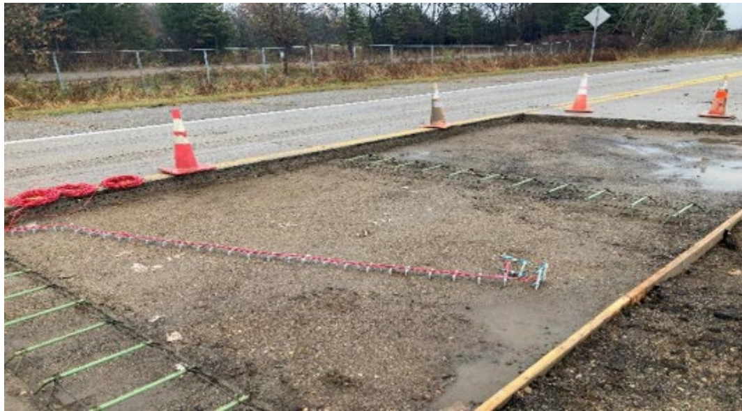
Figure 3.7 Picture accentuating sensor location and paving progression
