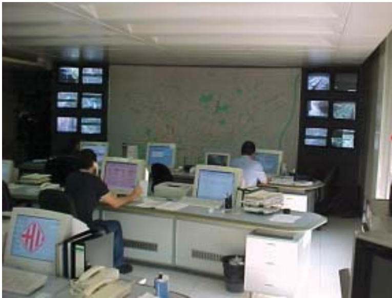
Figure 11. Barcelona City traffic management center.
