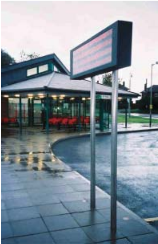
Figure 56. Ryton rural interchange, Newcastle.
