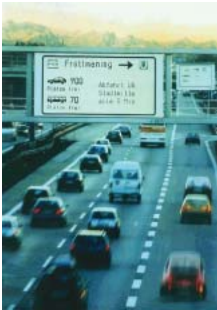
Figure 19. Multimodal dynamic message sign in Munich.
