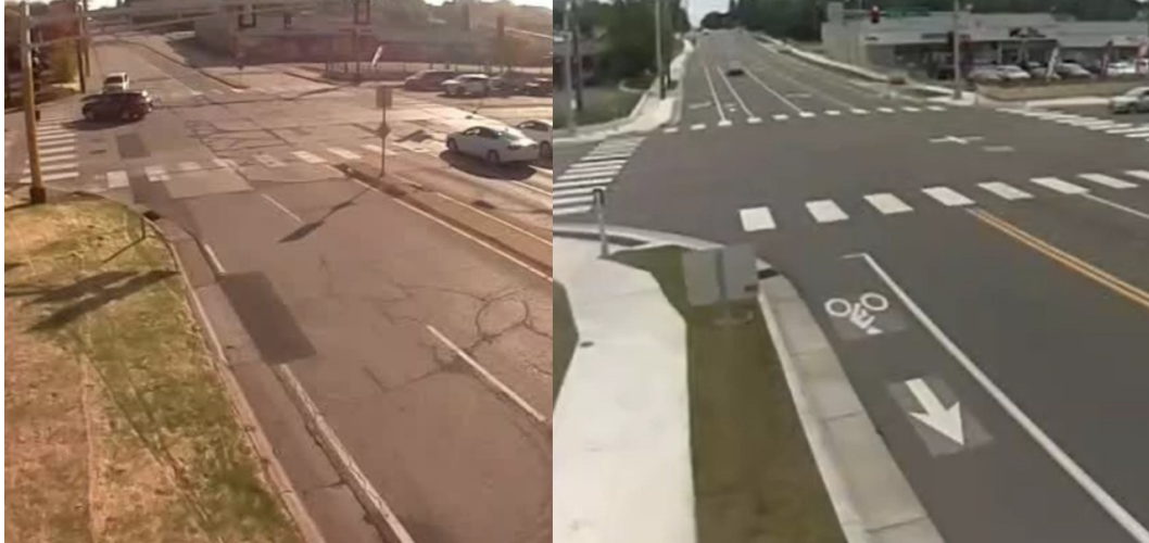
Figure 2.13 Image of Larpenteur from 2023 (left) and 2025 (right) with the car lane converted into a bicycle lane at the bottom of the image
