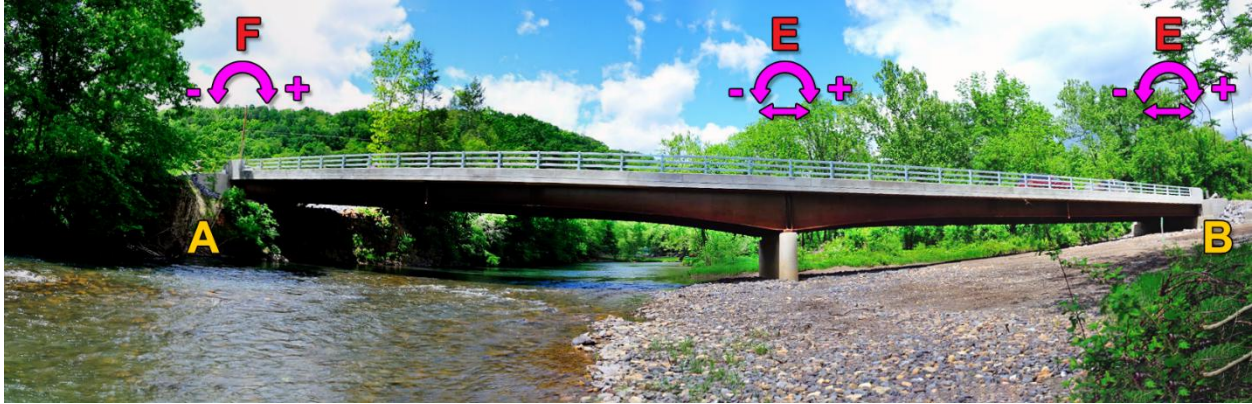
Figure 18. Photograph of In-Service Expansion and Rotation Diagram at Structure No. 29342. Curved and straight arrows indicate the direction of positive and negative rotation and displacement, respectively. A = Abutment A (full integral); B = Abutment B (semi-integral); E = expansion bearing; F = fixed bearing.
