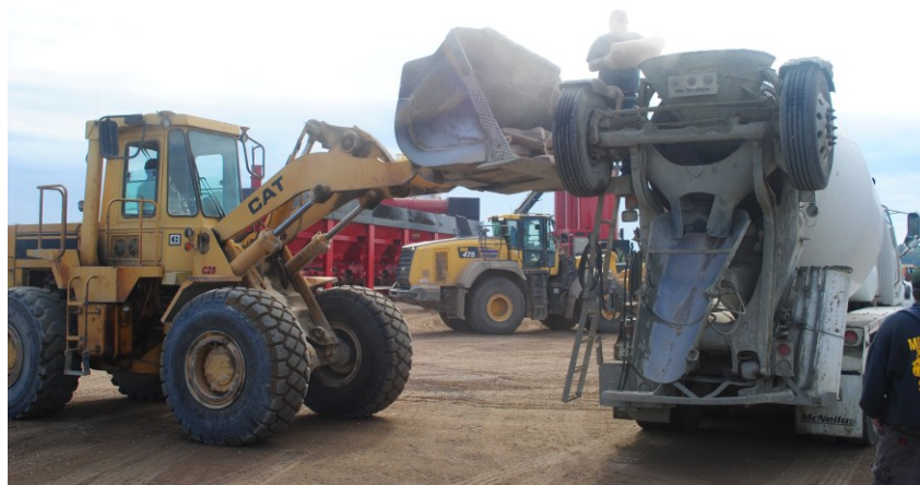
Figure 4.1 Mixing of treatment media in a concrete ready-mix truck.
