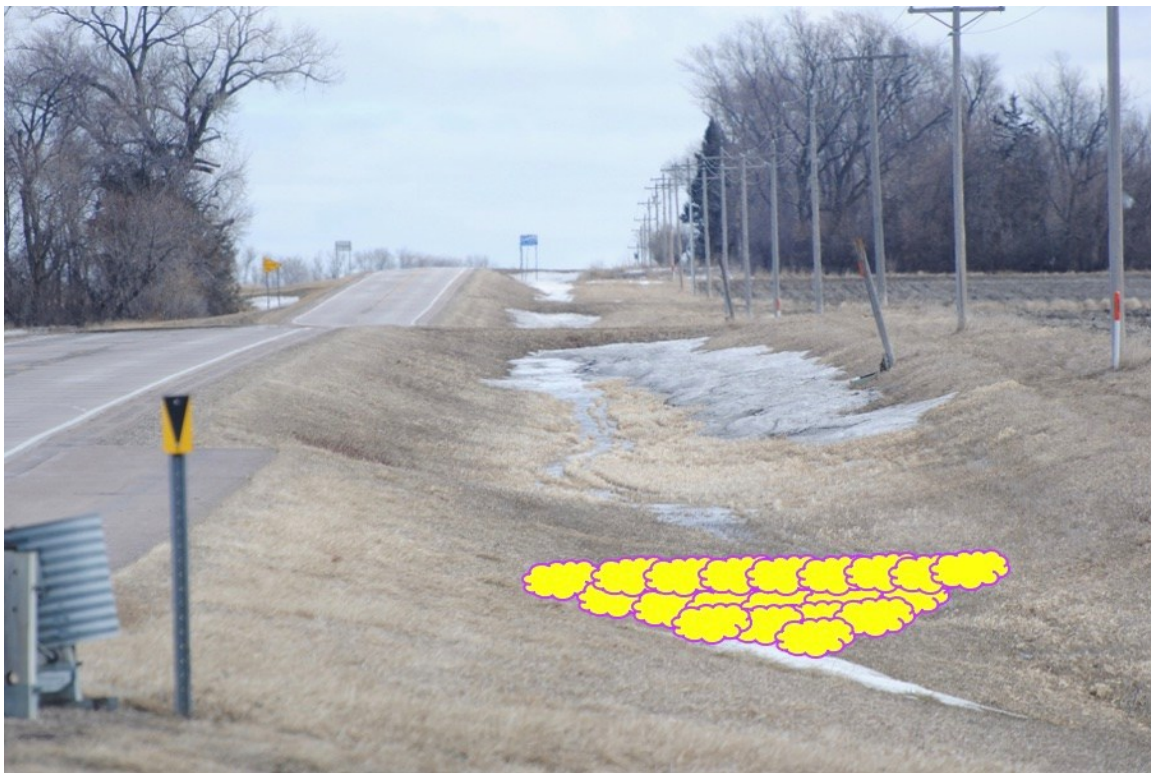
Figure 3.1 Illustration of a possible configuration of in-ditch treatment for salt capture, sketched onto an actual state highway drainage ditch during winter melt-out conditions.
