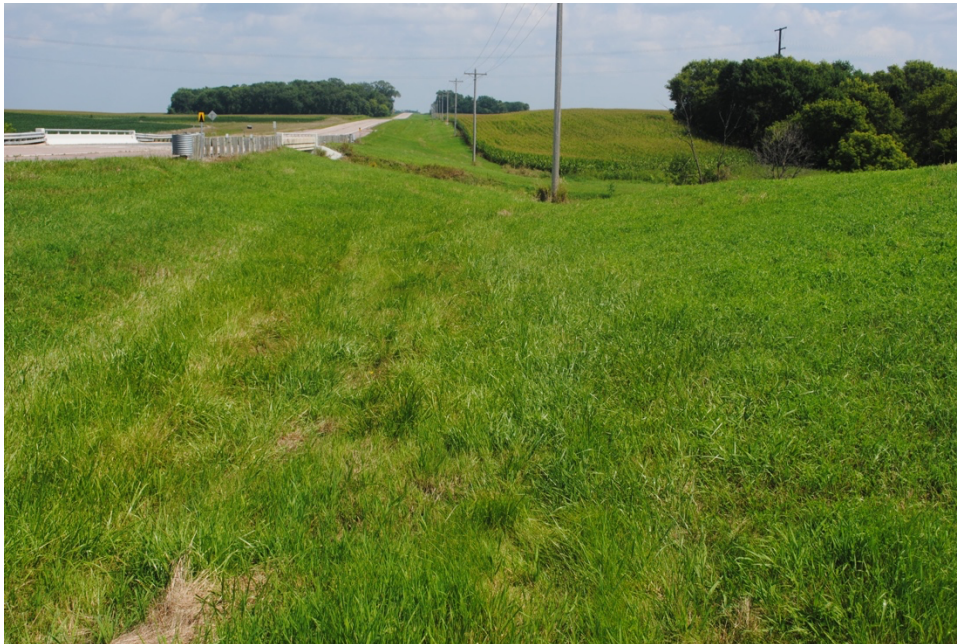
Figure 2. Willow Creek West Study Location: MN 30 about 5 miles west of Amboy. View east from eastbound side ditch line. Treatment media and instrument location proposed for space directly in front of camera location.
