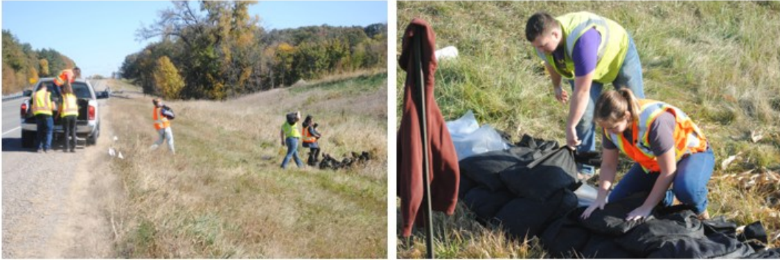
Figure 4.7 Treatment bag hauling to berm location (left); bag placement (right).
