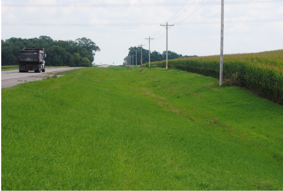
Figure 1. Willow Creek East Study Location: MN 30 about 5 miles west of Amboy. View east from eastbound side ditch line. Treatment media and instrument location proposed for space directly in front of second utility pole, approximately 500 feet from photographer location.
