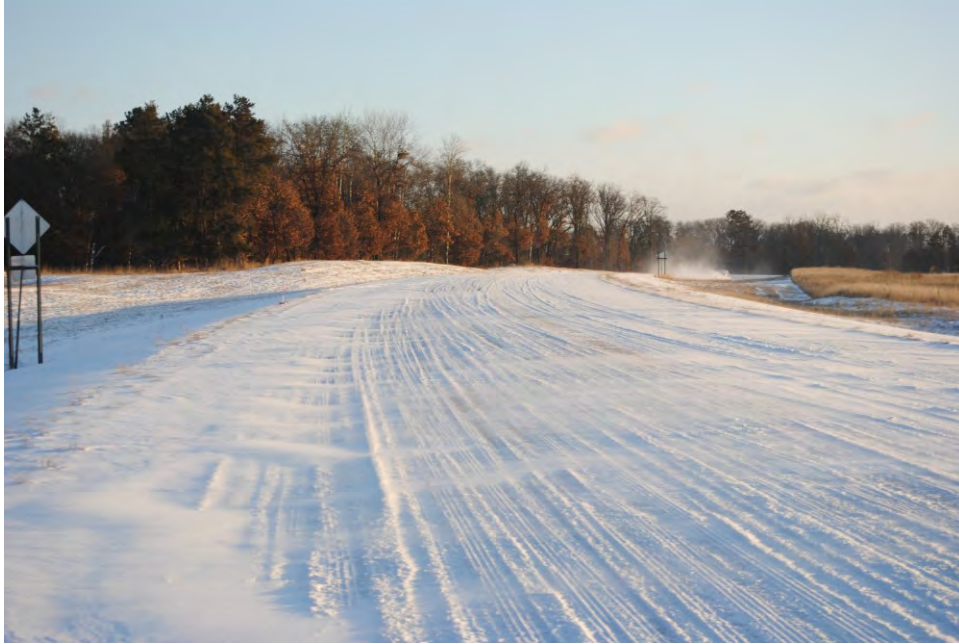
Figure 34. Perimeter track on testing day with compacted, frozen snow on the pavement.
