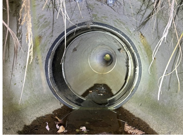
(b) Culvert 2225236, District 1: Elastomer Bands
