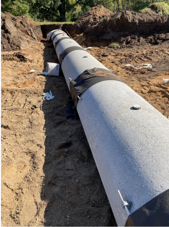
(a) Pipe prior to backfill
