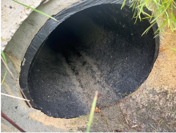
(a) Culvert 2231492, District 8: HDPE Liner
