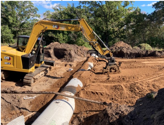
(c) Compaction of backfill
