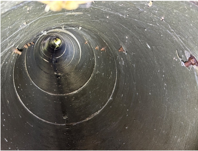
(a) Culvert 2207834 in District 8, Exterior Ties
