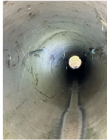
(b) Culvert 2183548 in District 2, Interior Ties
