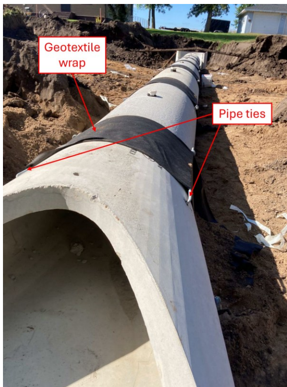
Figure 1.2: In-progress reinforced concrete pipe installation showing pipe ties and geotextile wrap
