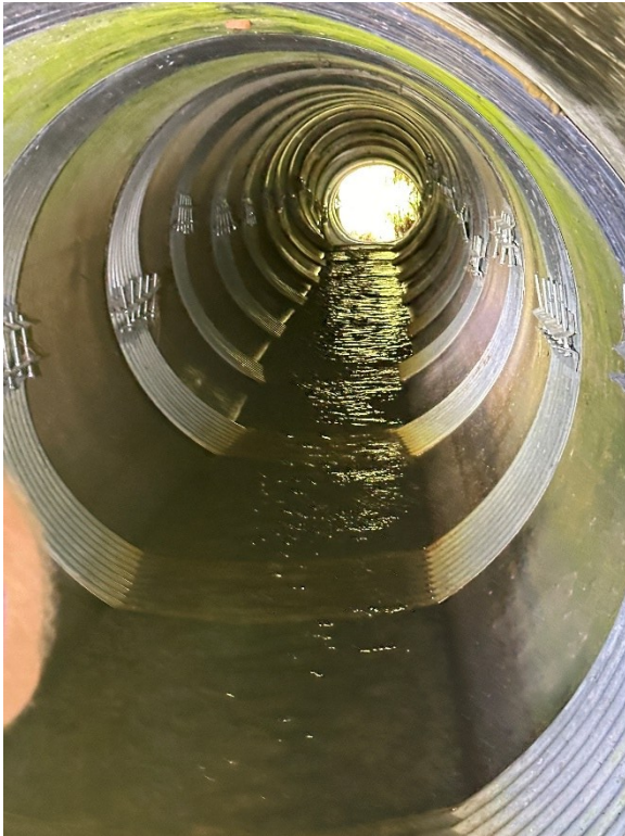
(c) Culvert 2214249, District 7: Metal bands
