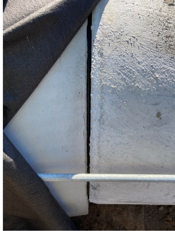
(b) Typical joint with mastic seal
