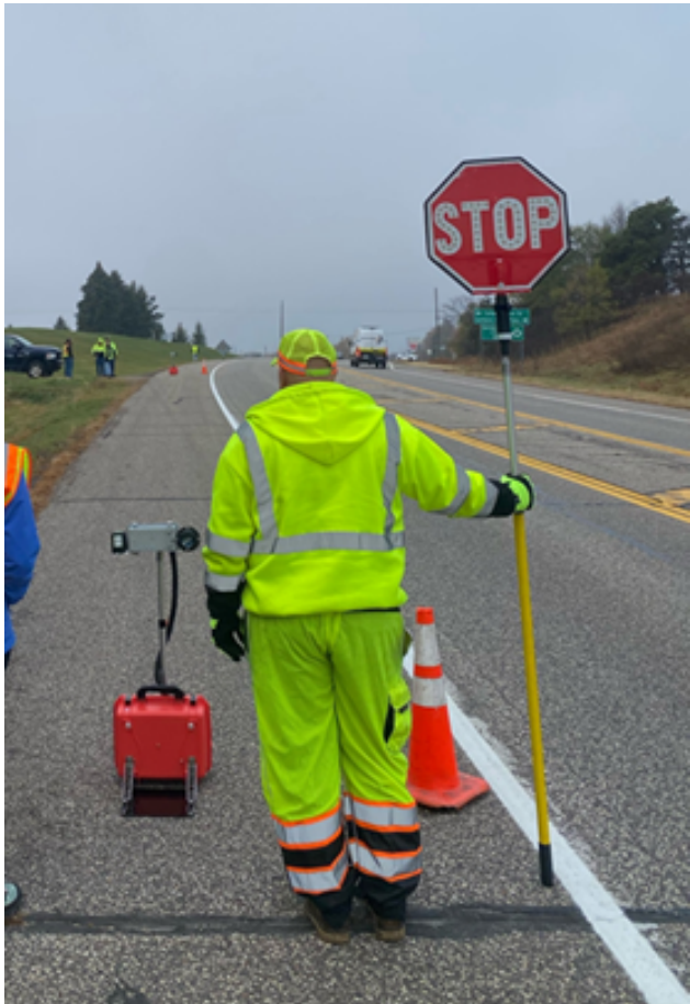
Figure 3.9 Pilot testing with the Washington County South Workshop in Woodbury.
