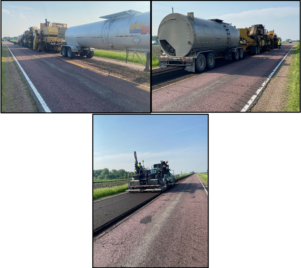
Figure B 7: CSAH 11 recycling train setup
