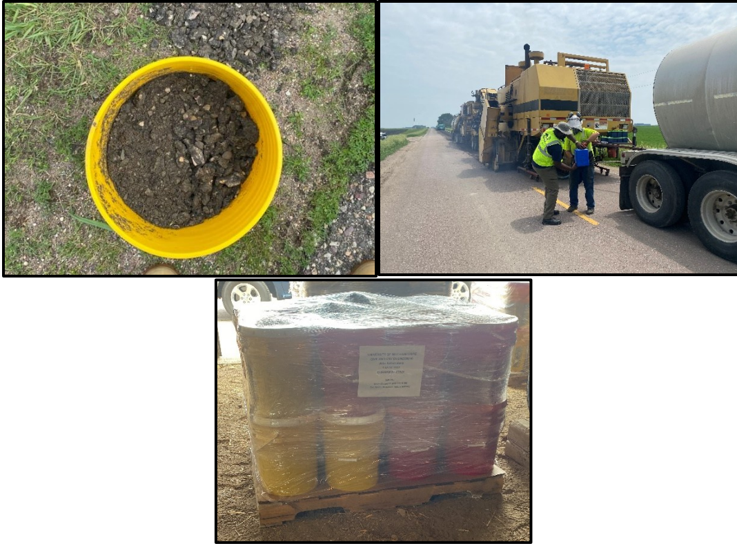
Figure B 17: CSAH 20 material sampling and storage/packaging
