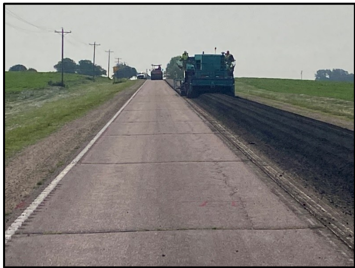
Figure B 19: CSAH 24 recycling train setup
