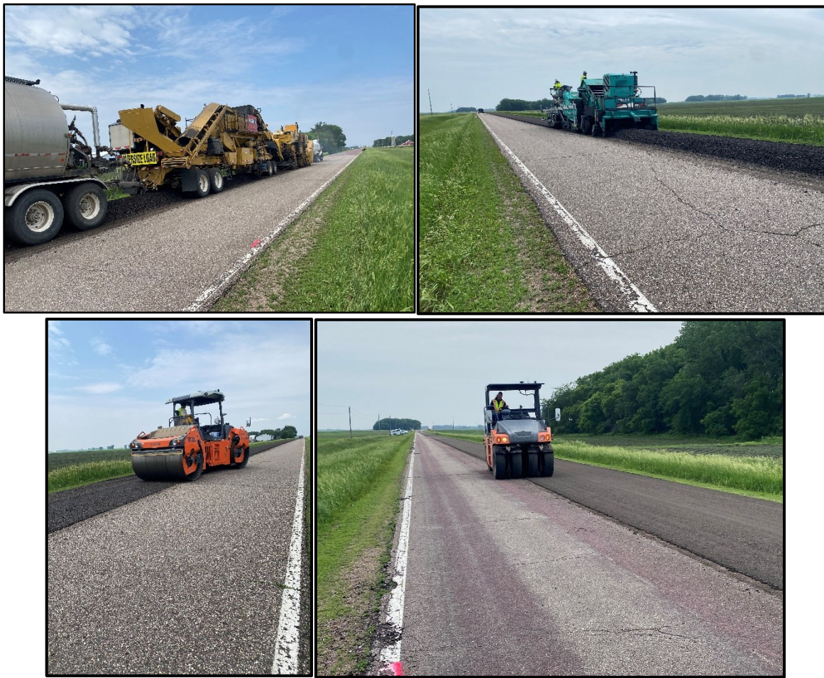
Figure B 14: CSAH 20 Recycling Train Setup
