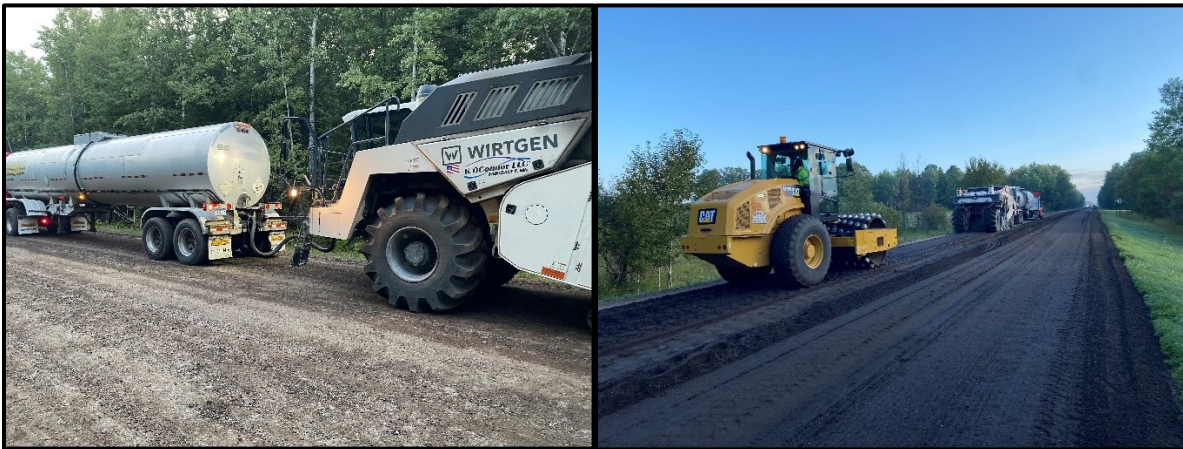
Figure B 2: CSAH 15 recycling train setup
