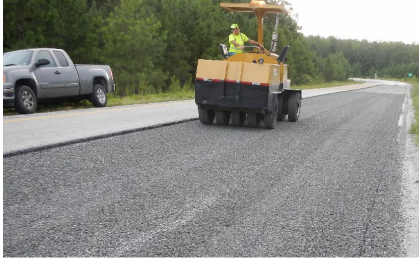
Figure 18. Pneumatic Roller.
