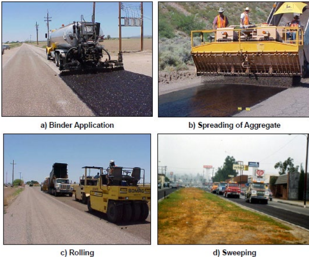
Figure 20. Construction process for chip seals (75).
