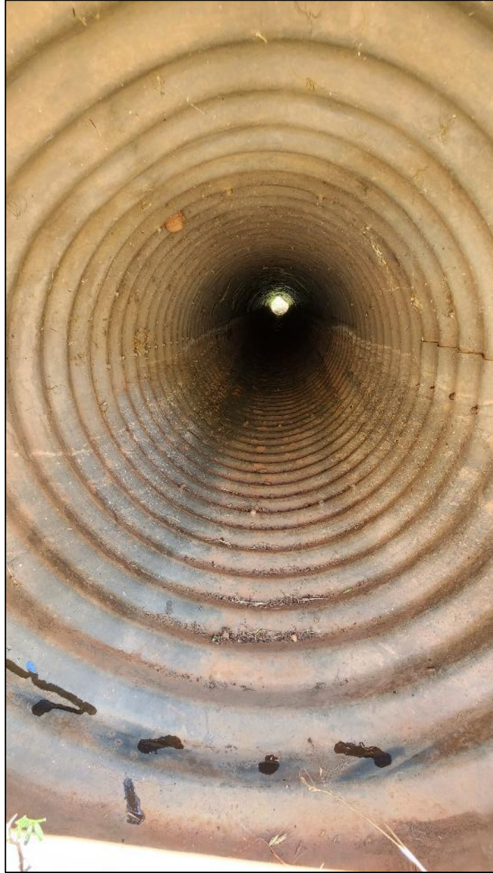
FIGURE 49: Culvert on NM 104 MP 42.1 inlet side looking in.
