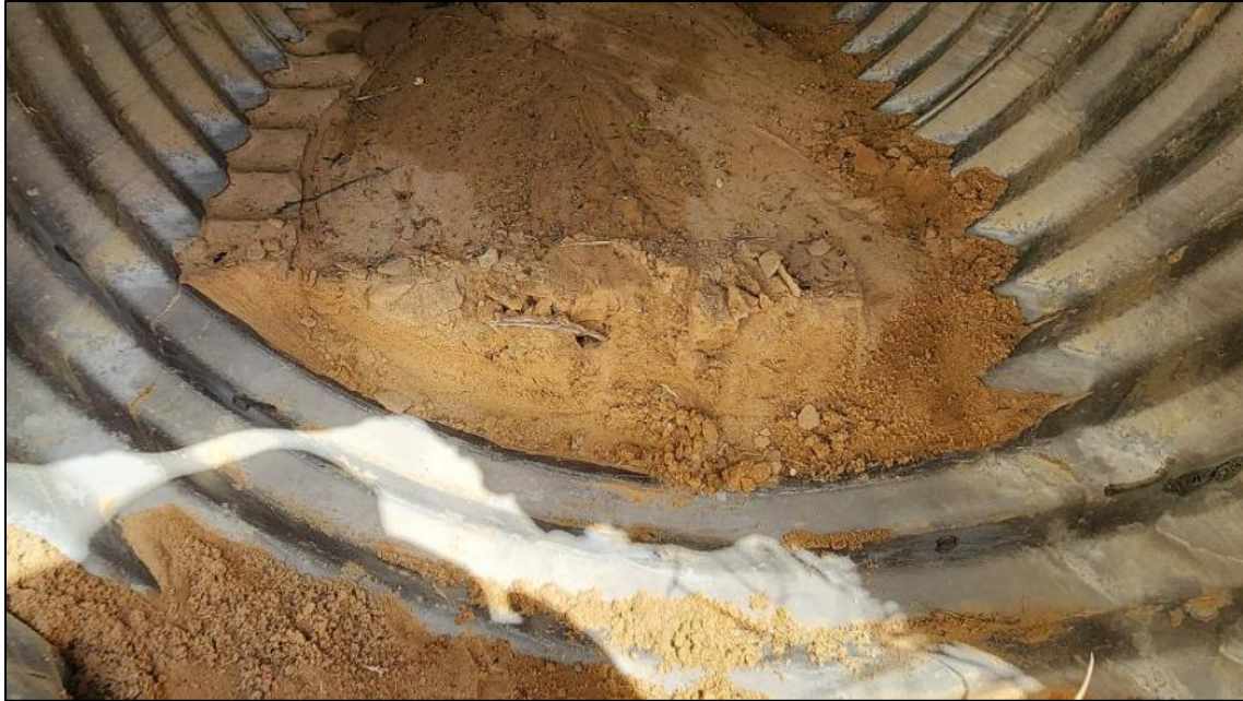
FIGURE 62: Location of ultrasonic thickness measurement, zero corrosion present, NM 117 MP 55 culvert.
