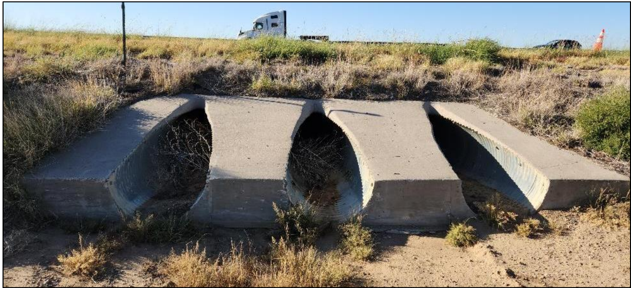
FIGURE 30: 3-36" CMP I-40 MP 121.0, inlet side, westbound I-40 (facing south).
