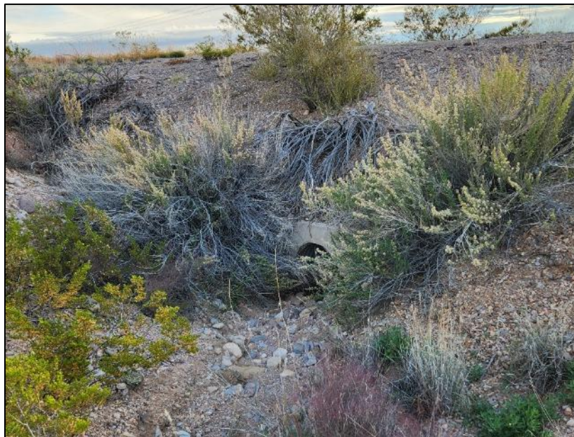
FIGURE 40: Inlet side of culvert on NM 1 MP 20.85.
