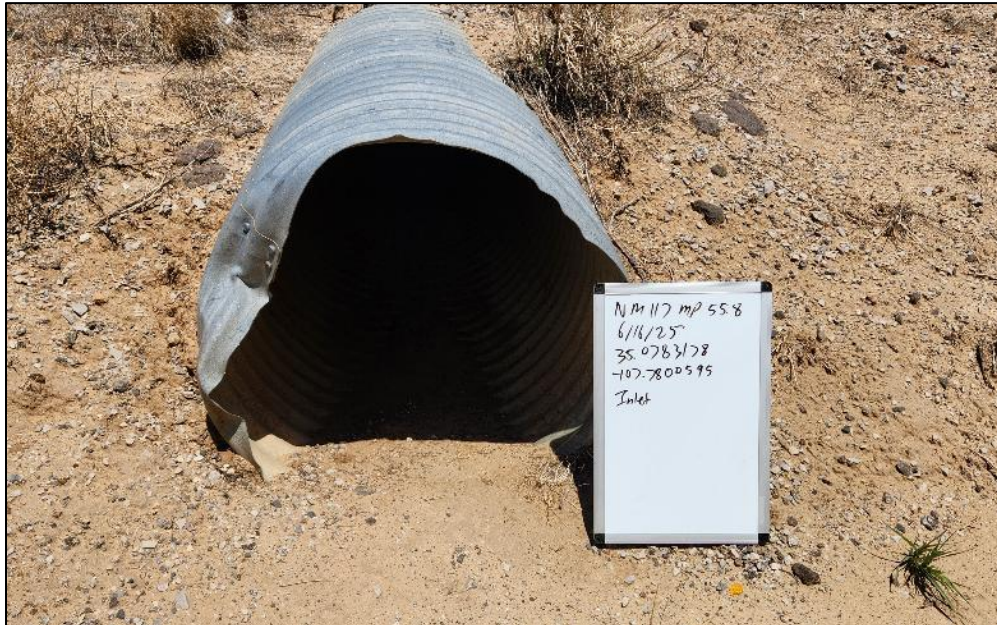
FIGURE 64: Culvert on NM 117 MP 55.8, inlet side.
