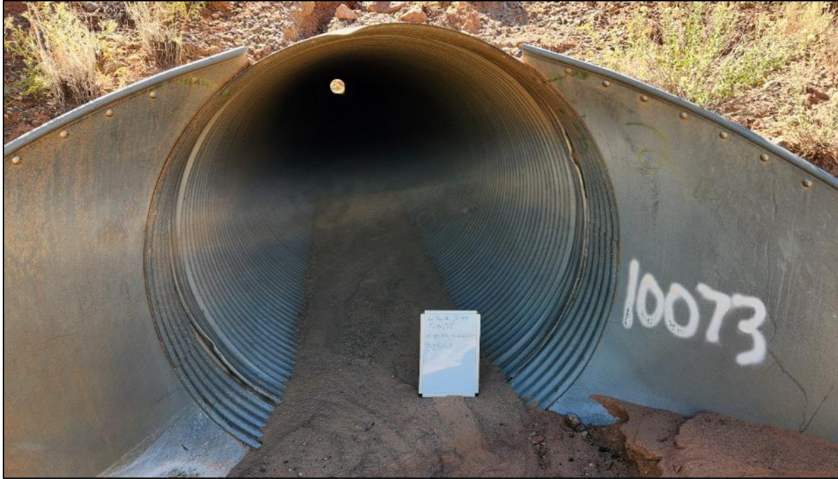
FIGURE 22: 72" culvert under I-25 at 264.2, inlet.
