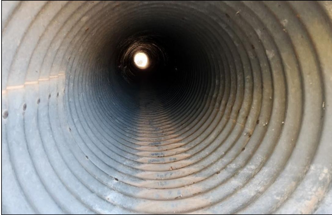
FIGURE 37: Inside of the inlet side of the culvert on NM 1 MP 19.24.
