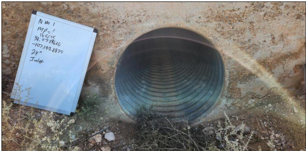
FIGURE 36: Culvert on NM 1 MP 19.24, inlet side.
