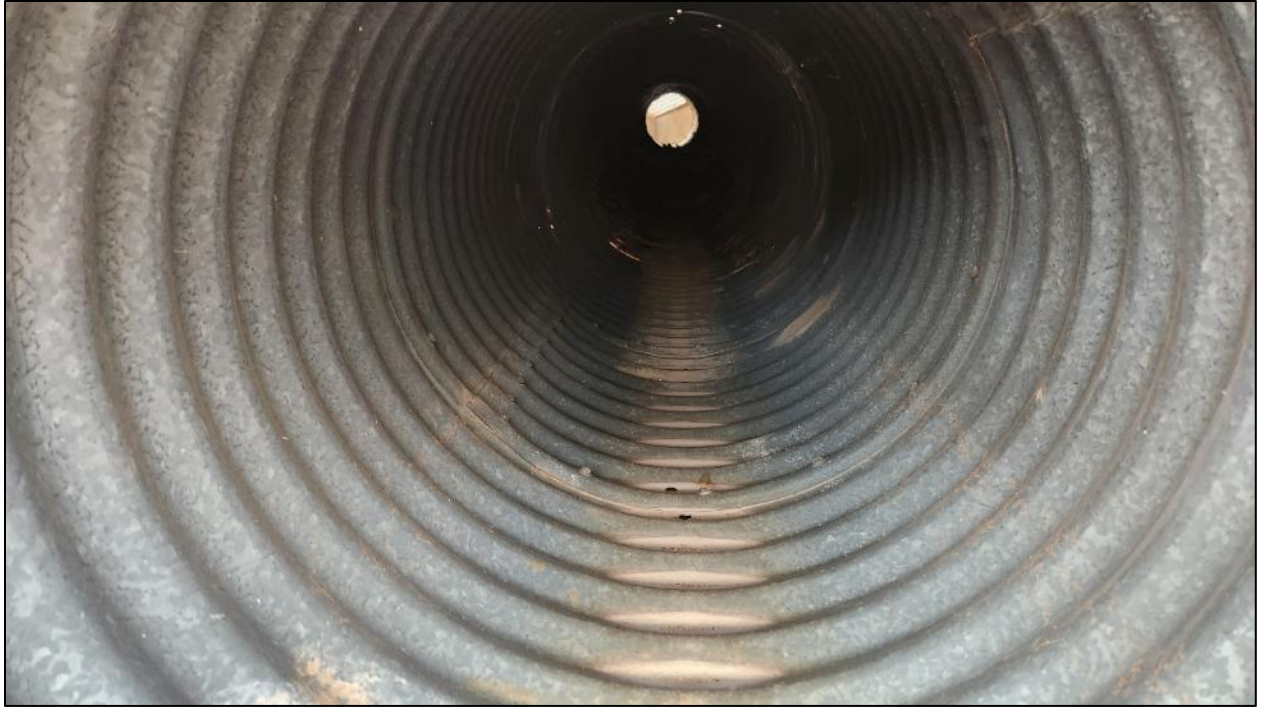
FIGURE 14: Culvert on I-25 (NB) MP 142.49, inside view near outlet side.
