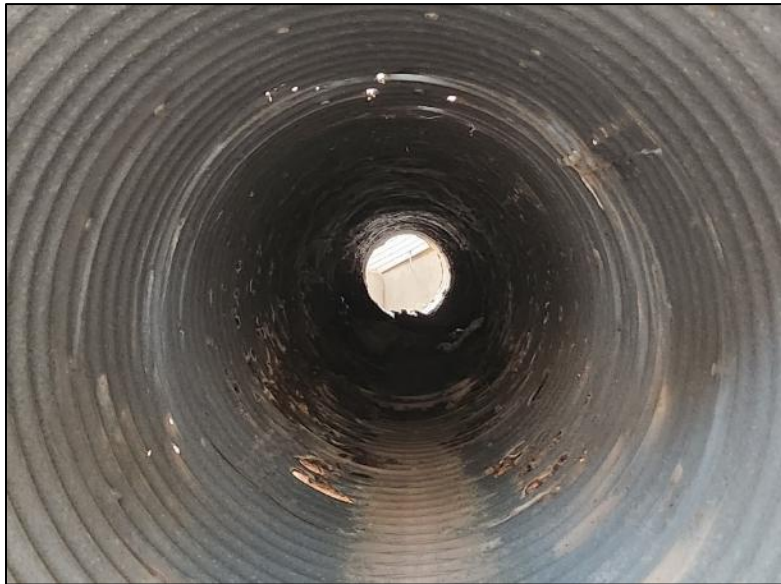
FIGURE 15: Culvert on I-25 (NB) MP 142.49.
