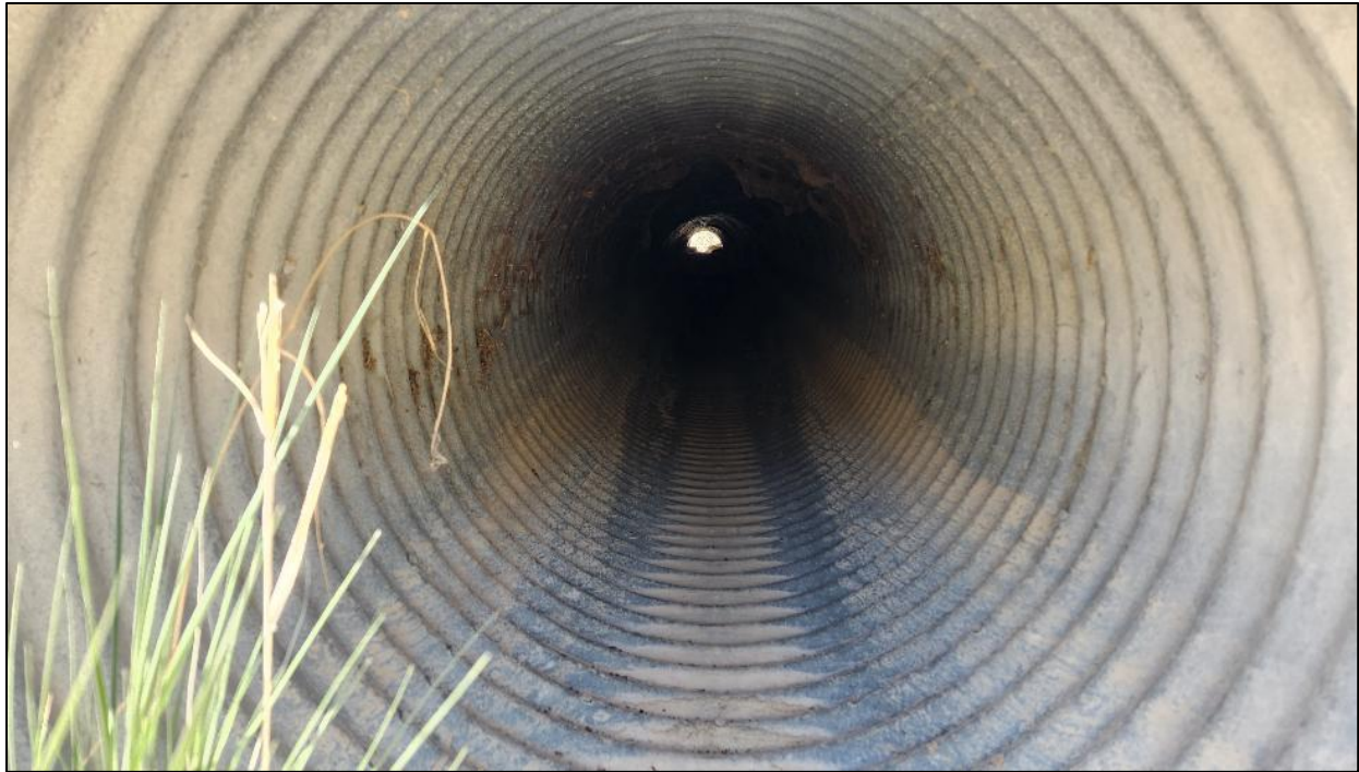
FIGURE 69: Culvert on NM 117 MP 56, close-up of inside on inlet side.
