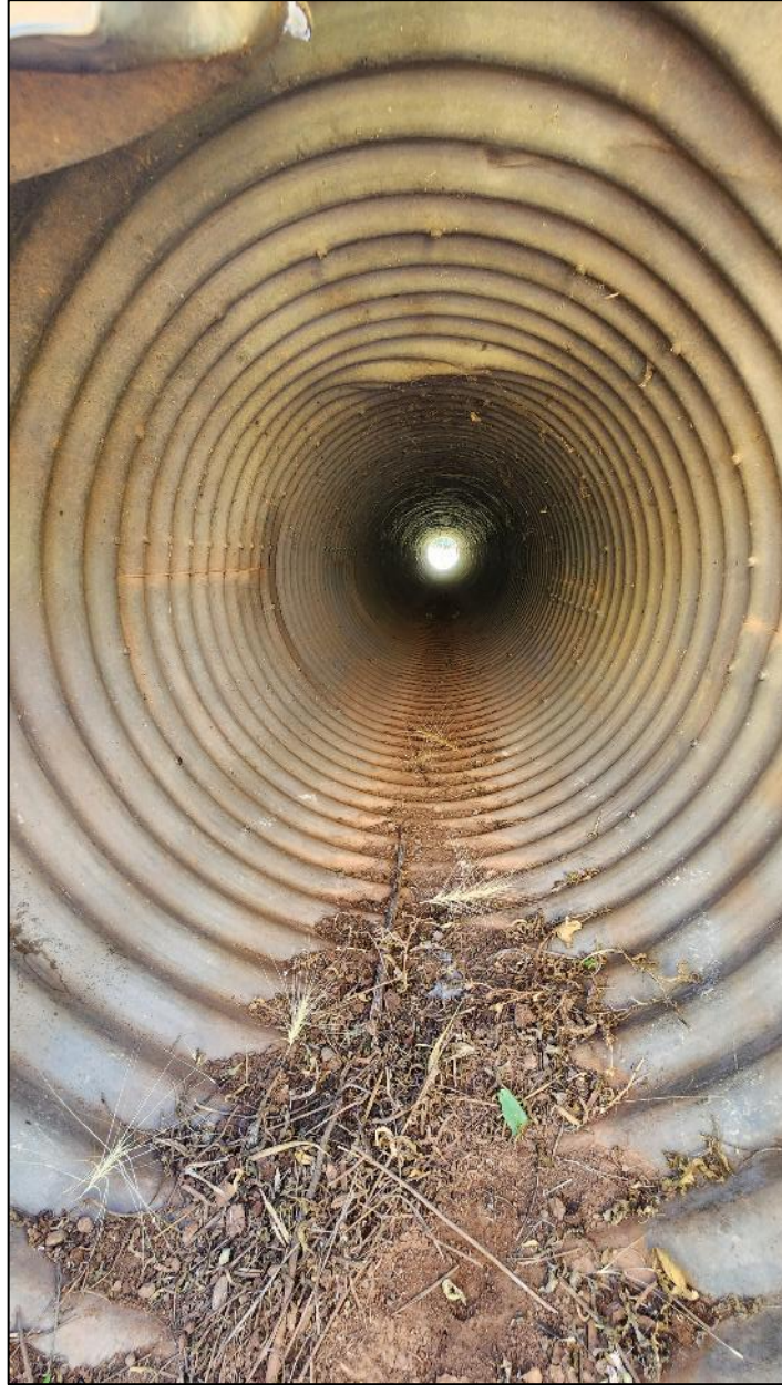
FIGURE 57: Culvert on NM 104 MP 46.9, inlet side looking in.
