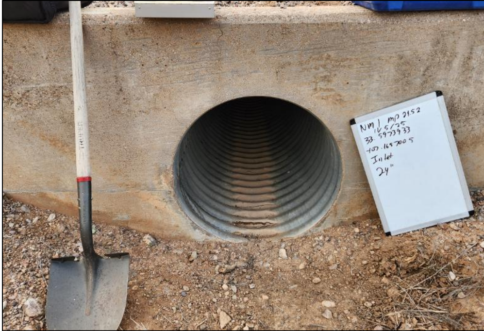
FIGURE 41: Culvert on NM 1 MP 21.52, inlet side.
