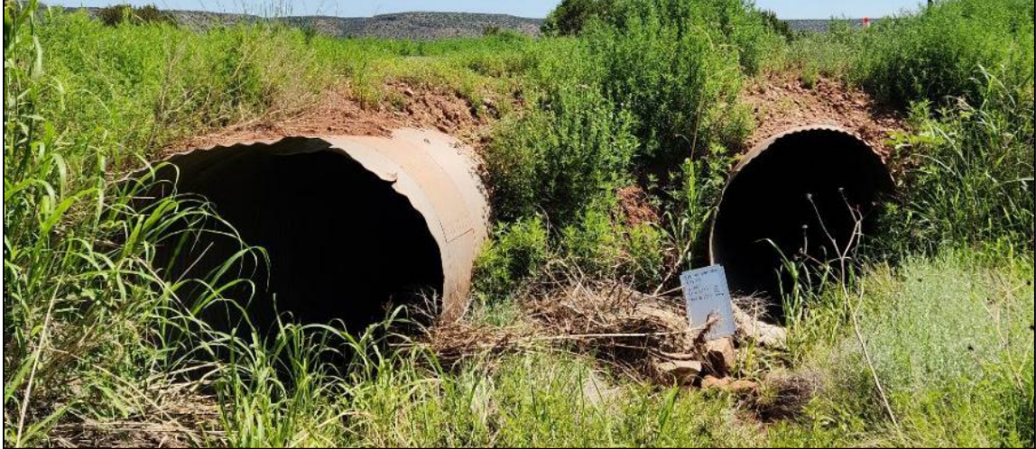
FIGURE 51: Two 60” culverts on NM 104 MP 43, inlet side.
