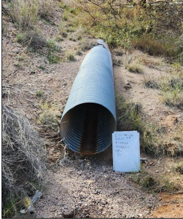
FIGURE 5: Culvert on I-25 (NB) MP 107.86, outlet side.
