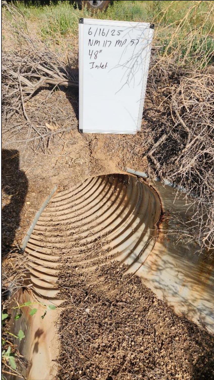
FIGURE 71: Culvert on NM 117 MP 57, inlet side.
