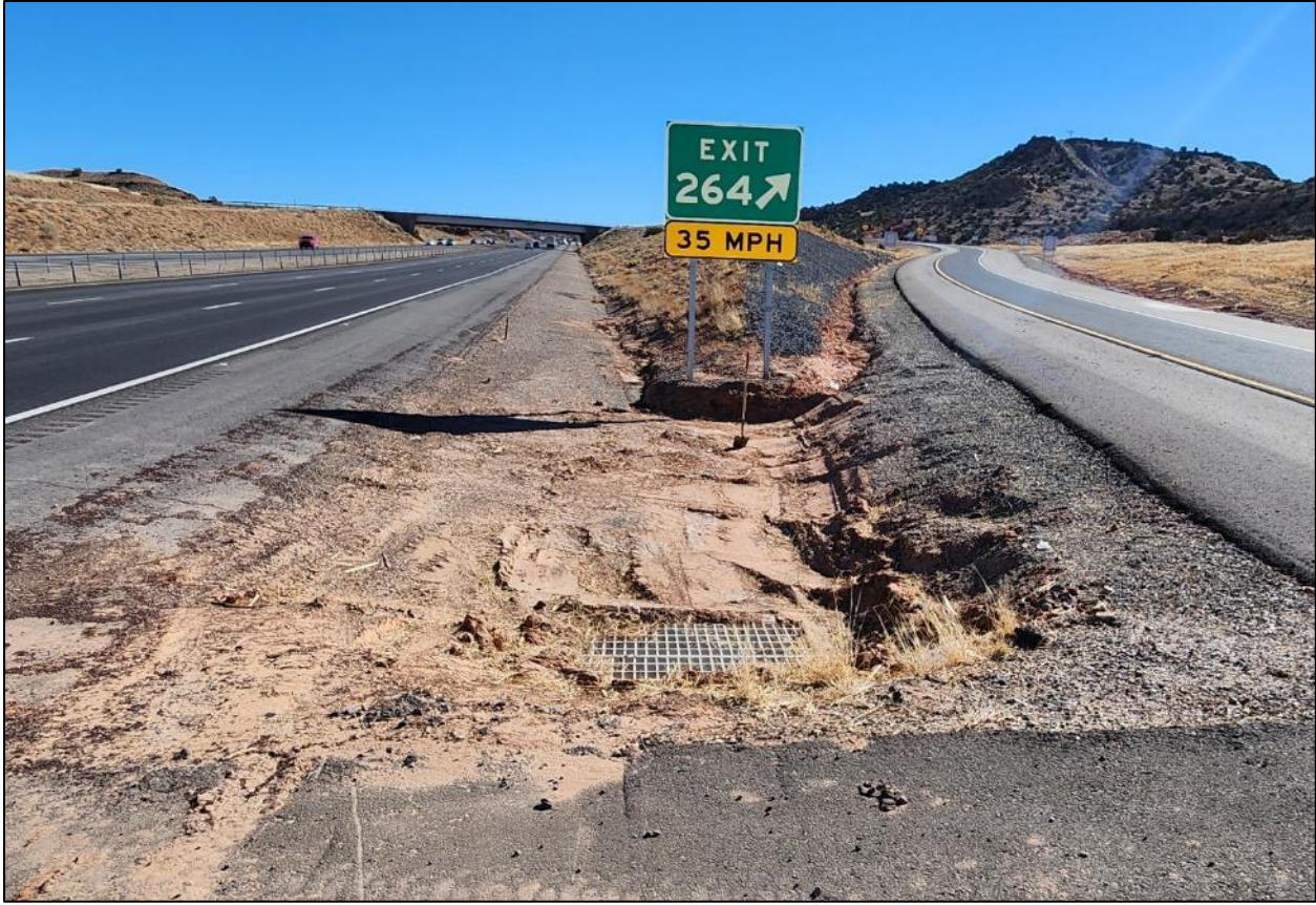
FIGURE 18: Image of “Inlet Grate” between NB I-25 and the offramp for exit 264.
