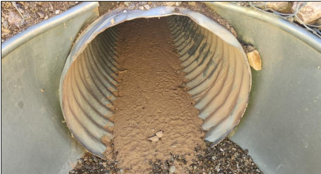
FIGURE 94: 24” culvert under NM 290, MP 1.0, inlet side facing south.
