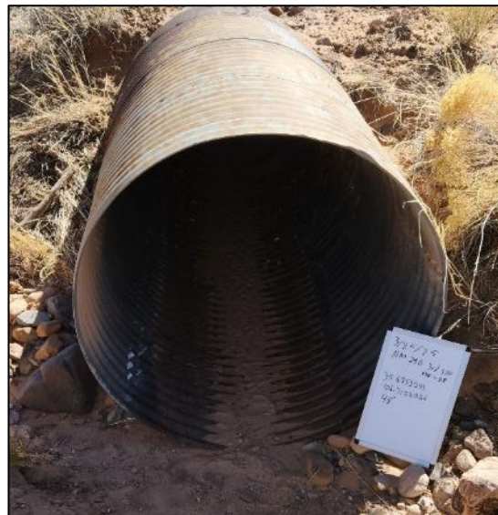
FIGURE 84: Culvert on NM 290 MP 0.65, inlet side.
