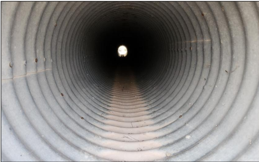
FIGURE 42: Inside of the inlet side of the culvert on NM 1 MP 21.52.
