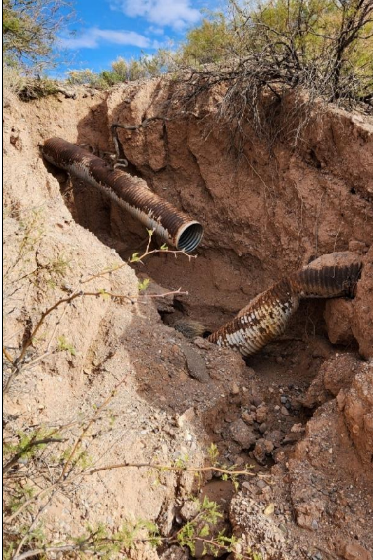
FIGURE 4: Culvert on I-25 (NB) MP 77.19.
