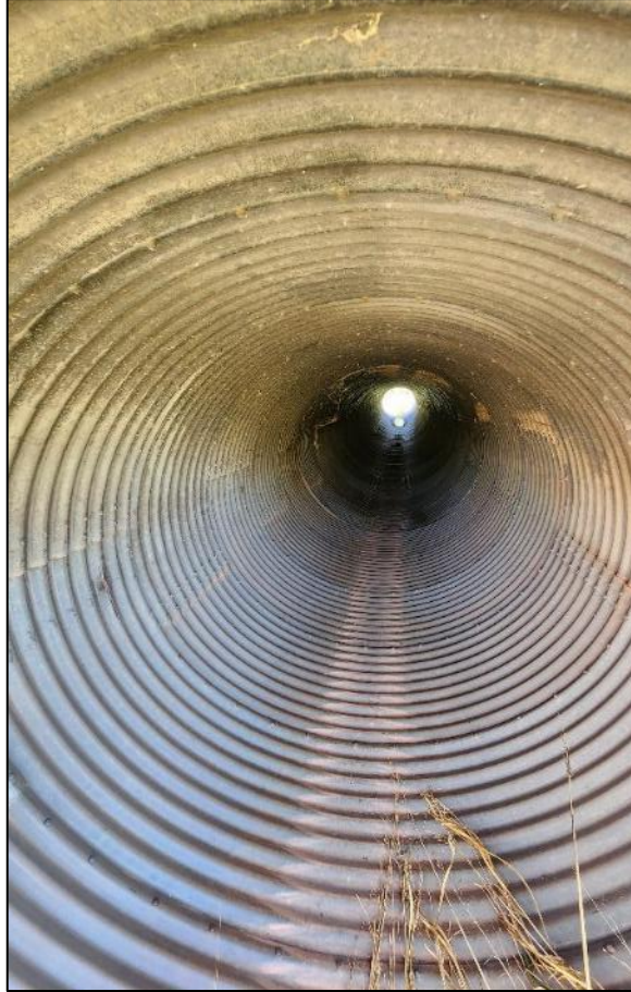
FIGURE 53: Eastern 60” culvert on NM 104 MP 43, inlet side looking in.
