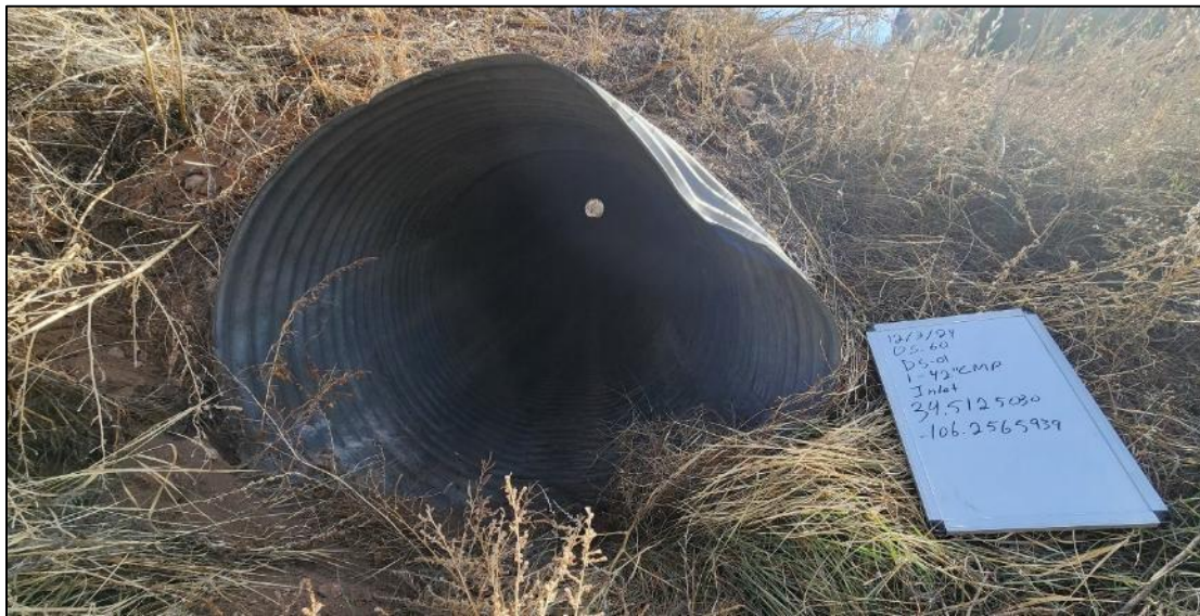
FIGURE 97: 42” culvert under US 60 MP 203.41, inlet side facing south.
