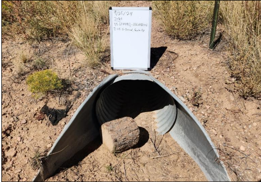
FIGURE 27: Culvert at I-25 (SB) MP 278.7, inlet side facing North.
