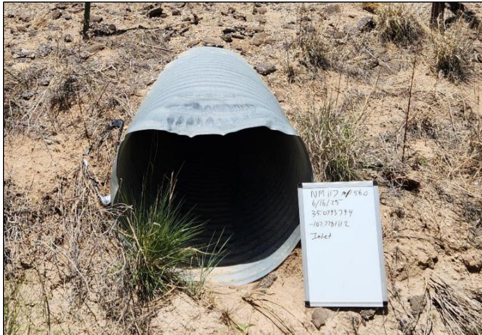
FIGURE 68: Culvert on NM 117 MP 56, inlet side.
