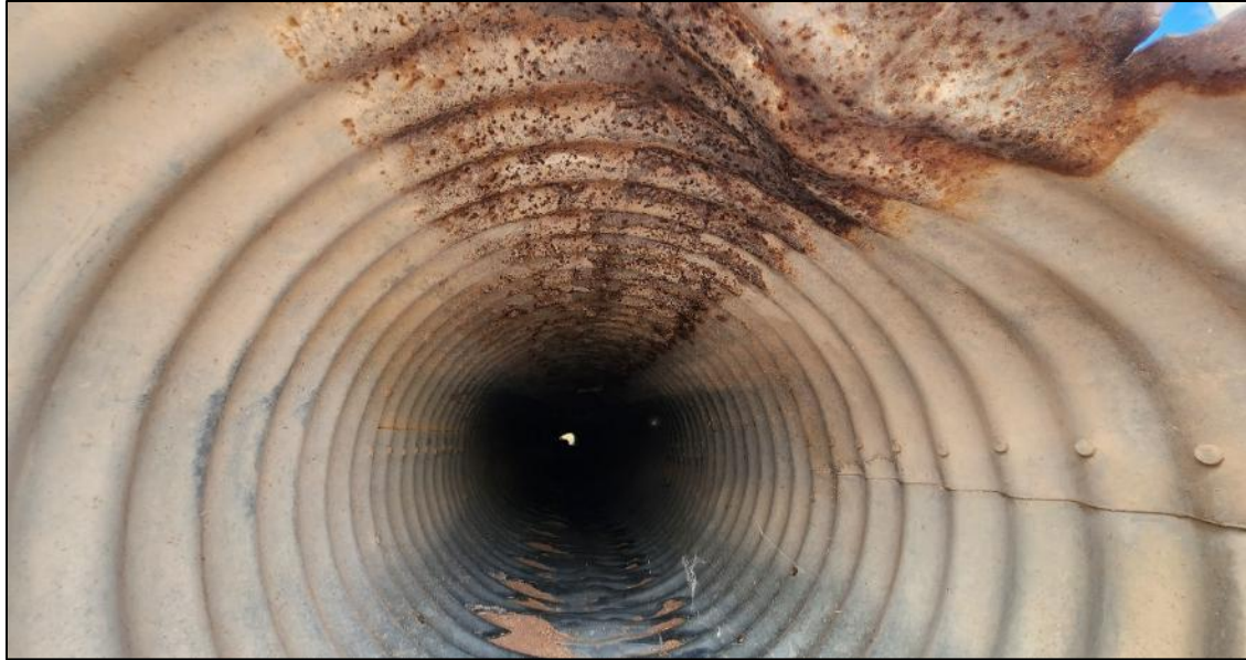
FIGURE 82: Inside of the inlet side of the culvert on NM 195 MP 1.51.
