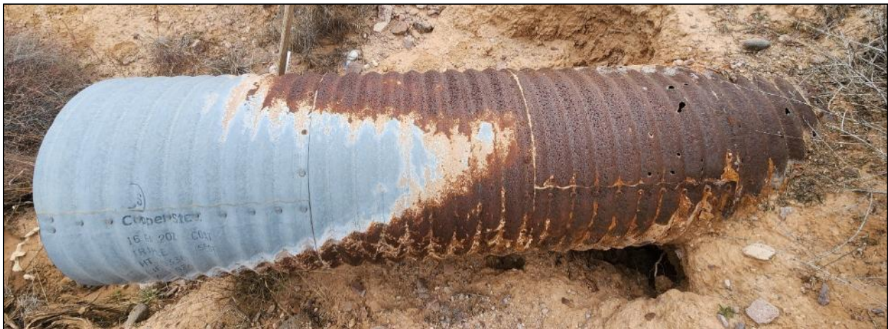
FIGURE 13: Culvert on I-25 (NB) MP 142.49, outlet side.
