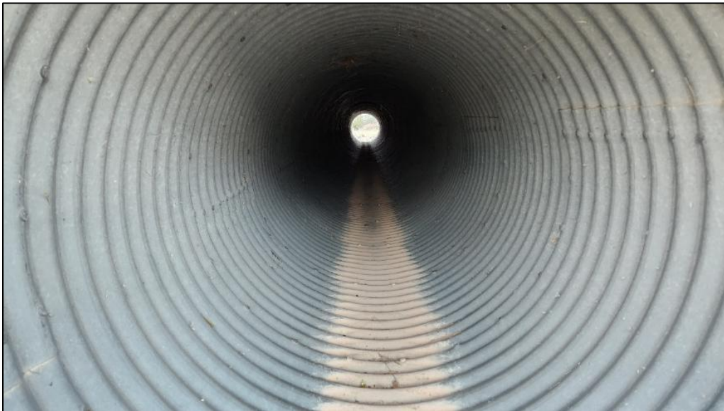
FIGURE 45: Inside of the inlet side of the culvert on NM 1 MP 22.01.
