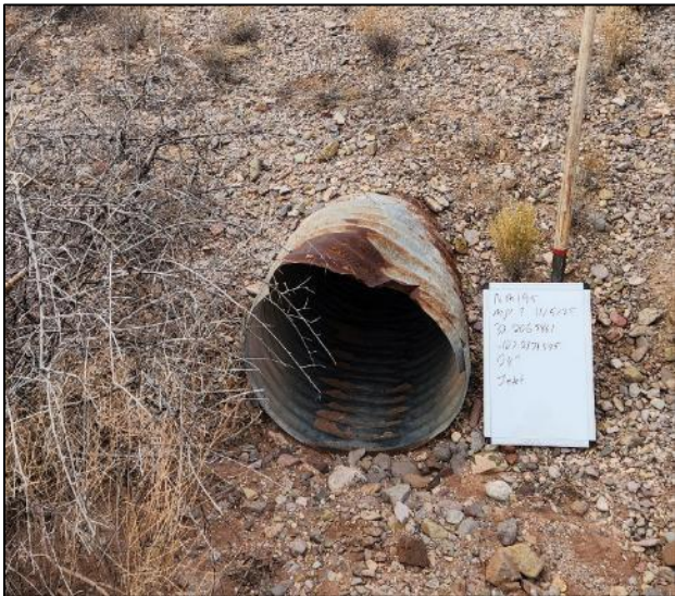
FIGURE 81: Culvert on NM 195 MP 1.51, inlet side.
