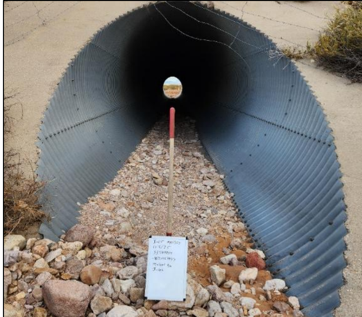
FIGURE 9: Culvert on I-25 MP 113.04, inlet side.
