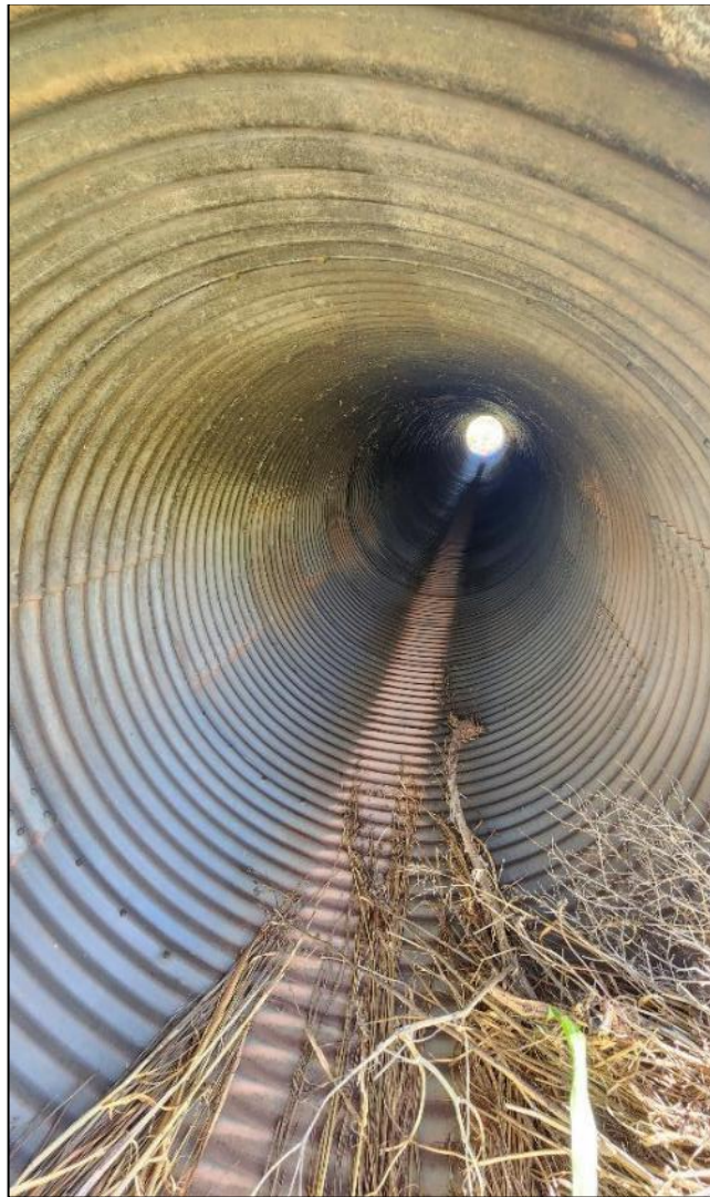
FIGURE 52: Western 60” culvert on NM 104 MP 43, inlet side looking in.
