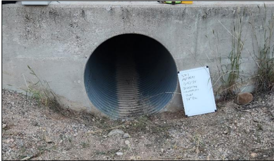
FIGURE 44: Culvert on NM 1 MP 22.01, inlet side.
