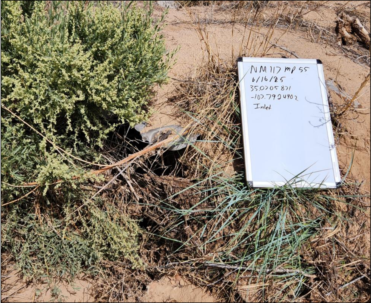
FIGURE 59: Culvert on NM 117 MP 55 inlet before removal of brush.
