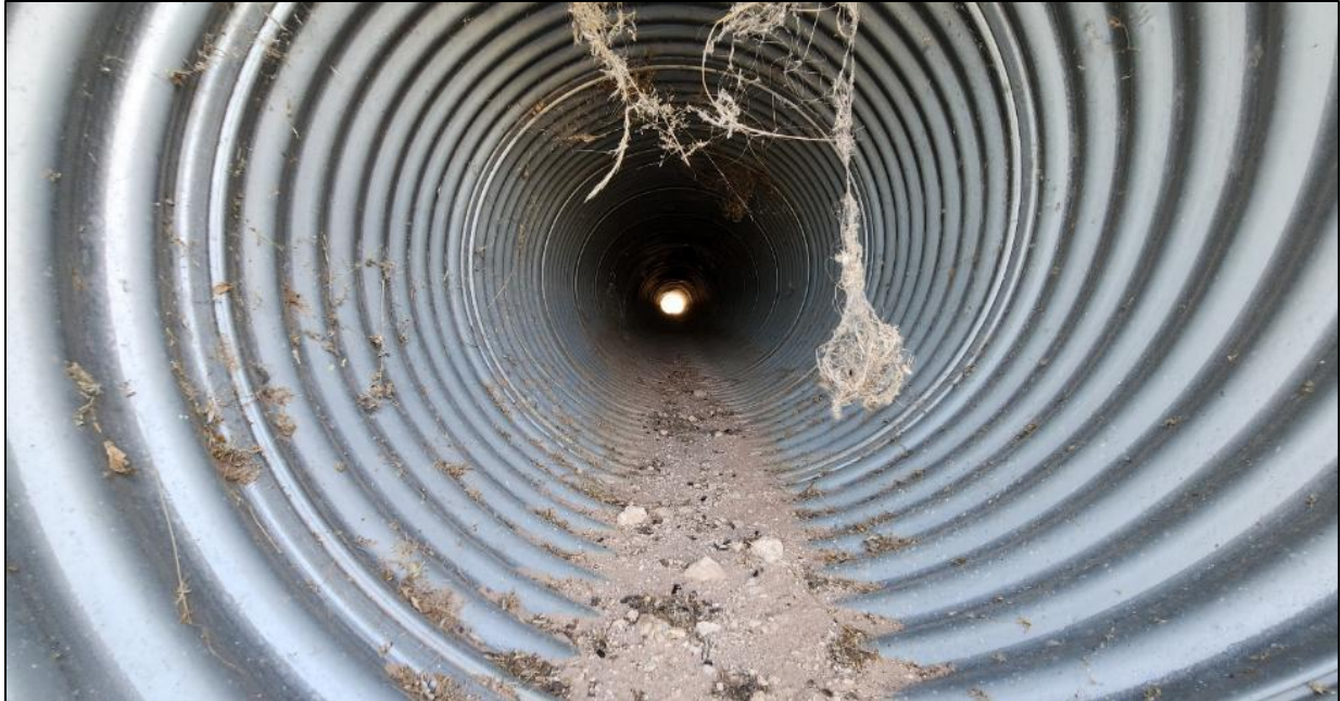
FIGURE 77: Western 36" culvert on NM 128 MP 21.93 facing south at inlet.
