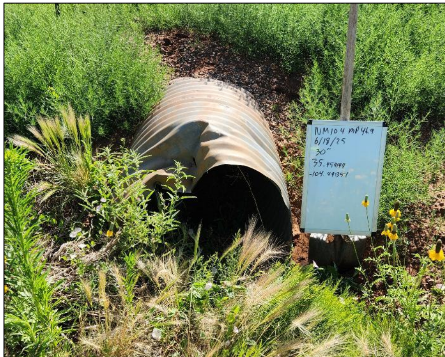
FIGURE 56: Culvert on NM 104 MP 46.9, inlet side.
