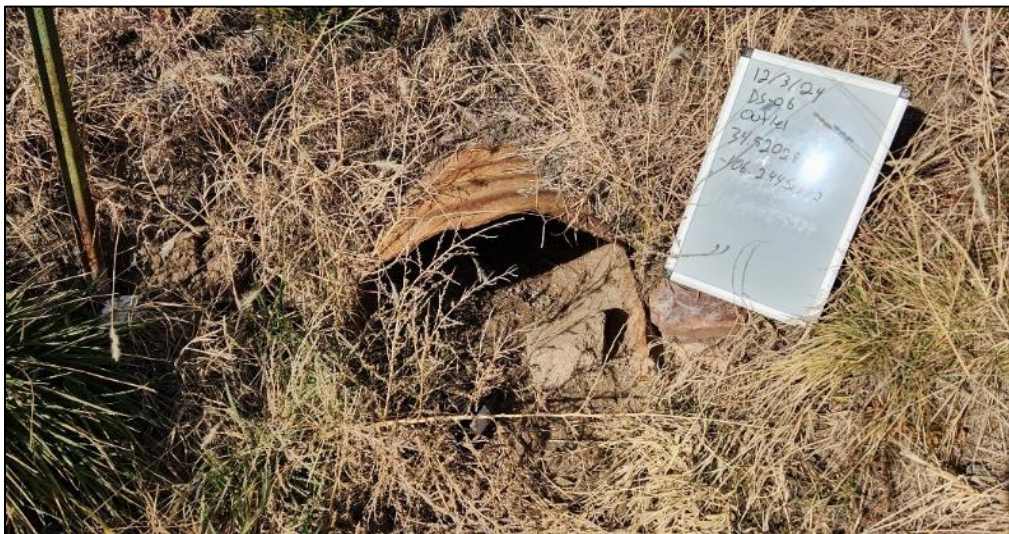
FIGURE 100: 24” culvert under US 60 MP 204.33, outlet side facing north.
