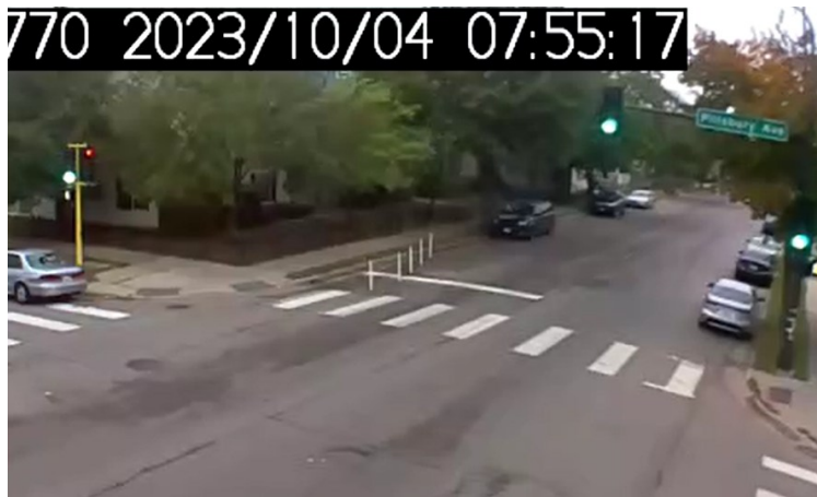
Figure 4.11 The first day of post-installation camera data at Pillsbury & 31st. Note the absence of the parked cars, replaced by the bollard curb extension.
