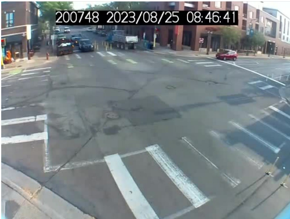
Images of Nicollet & 26 th , pre-installation (top image) and post-installation (bottom image).
