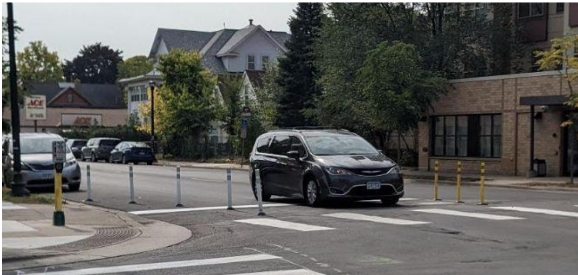
Figure 2.3 An example of a temporary curb extension and hardened centerline, located at Bloomington & 24th.
