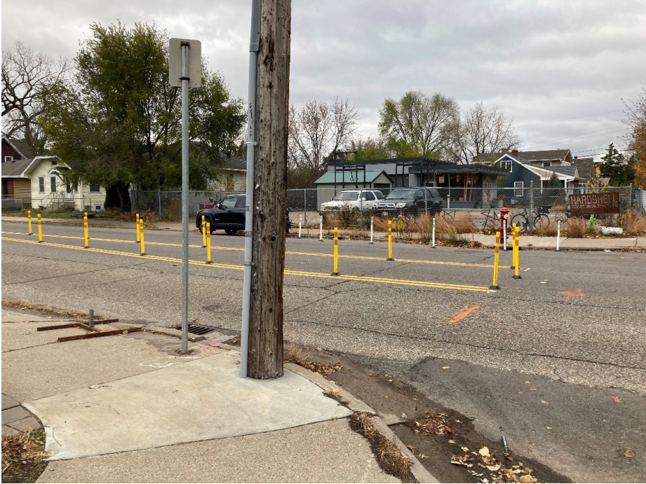
Figure 2.6 An example of a temporary pedestrian refuge, located at Longfellow Ave & E 38th St.
