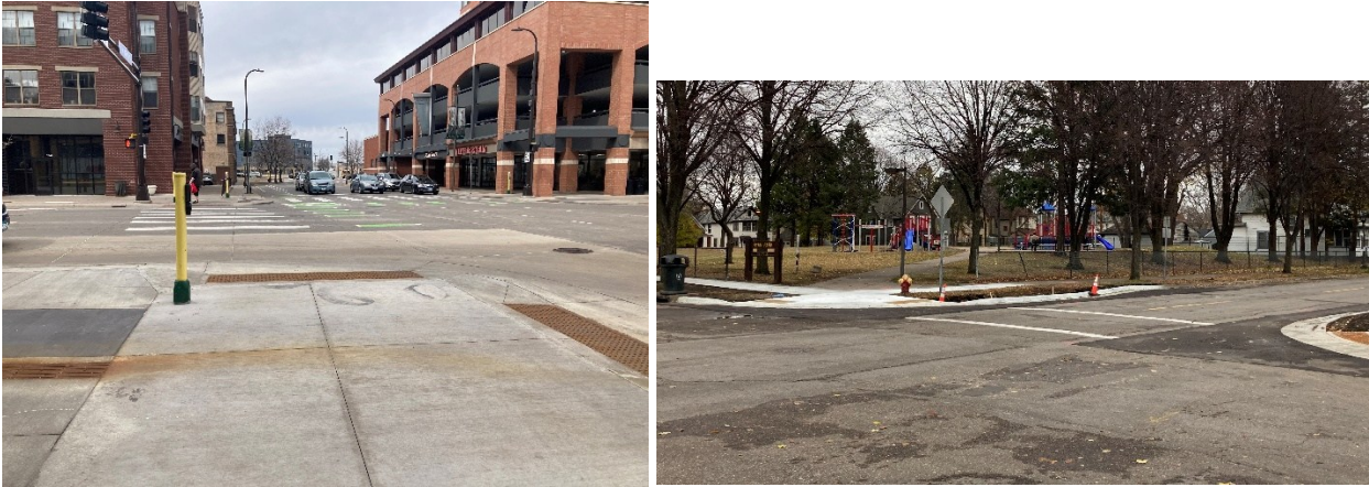
Figure 2.7 An example of a permanent curb extensions, located at N 12th St & Hennepin Ave (left), and N Avon St & Thomas Ave (right).
