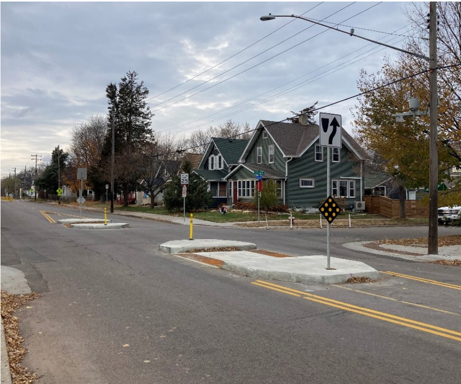
Figure 2.8 An example of a permanent pedestrian refuge, located at 22nd Ave S & E 35th St.
