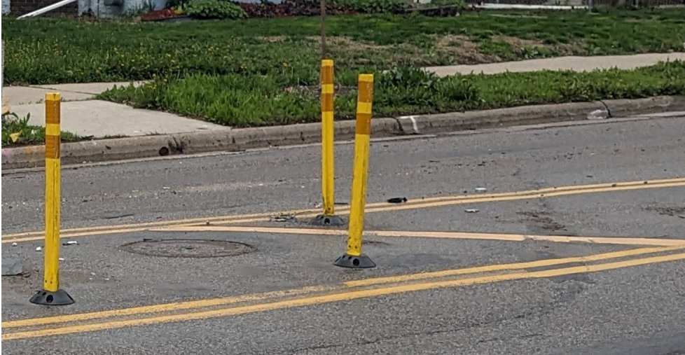
Figure 1.2 Image of a flexible delineator or bollard in yellow plastic with retroreflective markings/tape at the top of the post. Similar delineators are made in white and orange colors.
