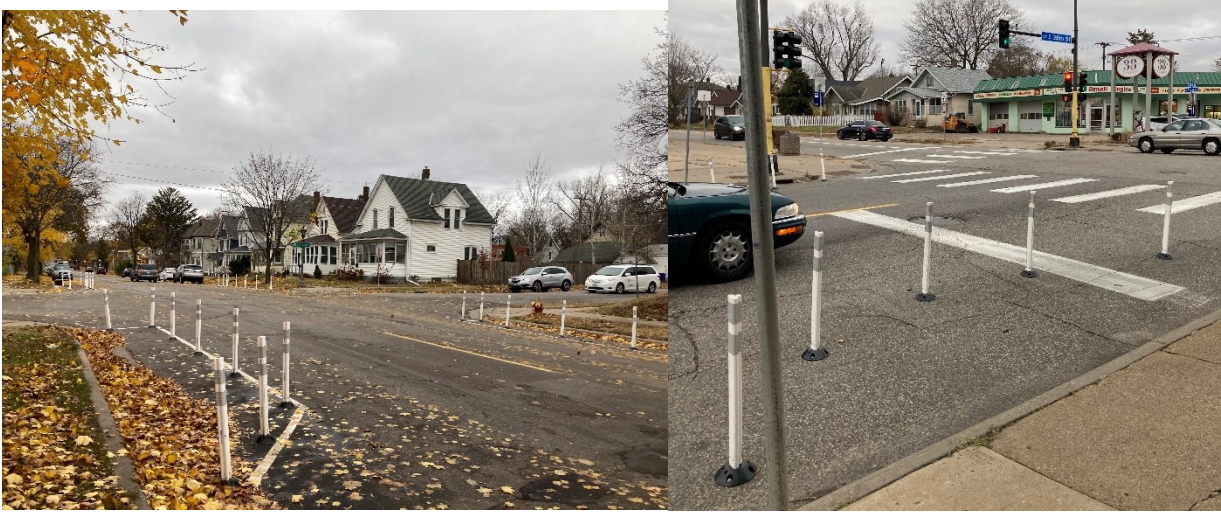
Figure 2.5 An example of a temporary curb extension, located at Milton St & Thomas Ave (left) and Cedar Ave S & E 38th St (right).
