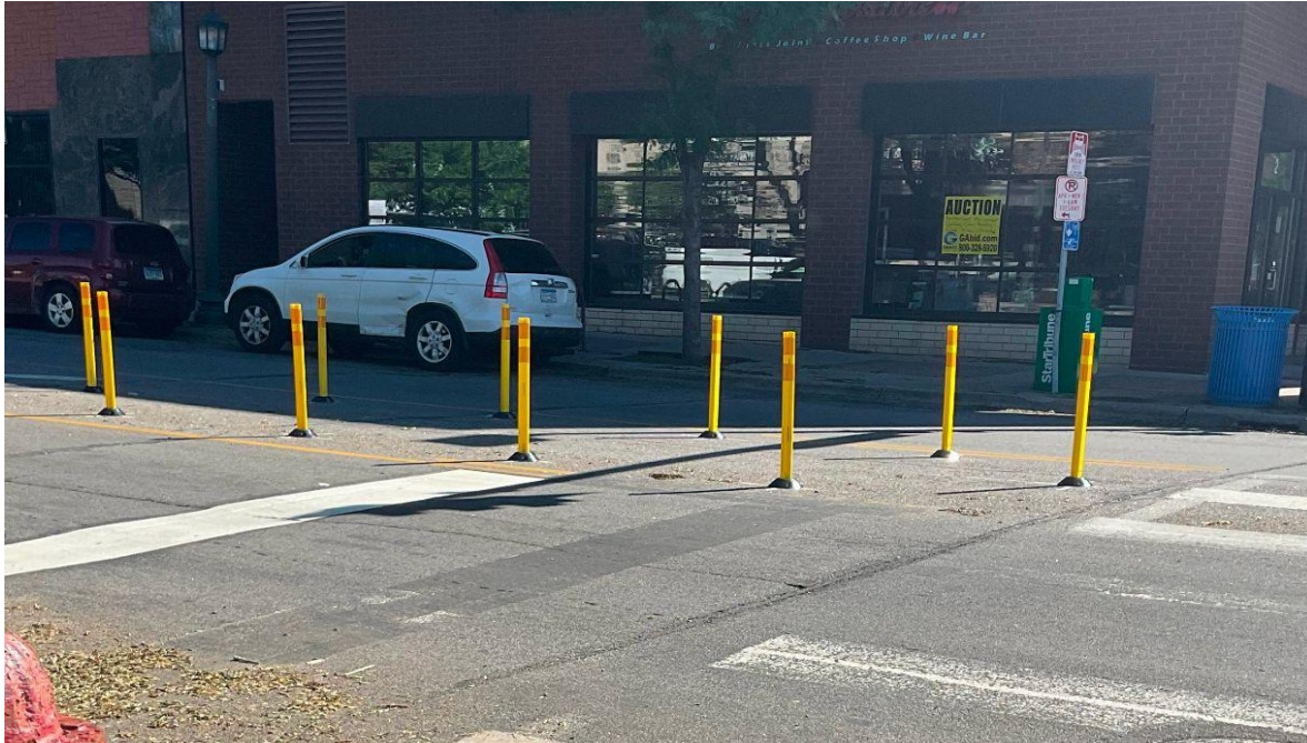
Figure 2.4 An example of a temporary pedestrian refuge or median, located at Nicollet & 26th.
