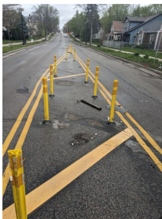
Figure 5.1 Temporary refuge section with bollards and paint.
