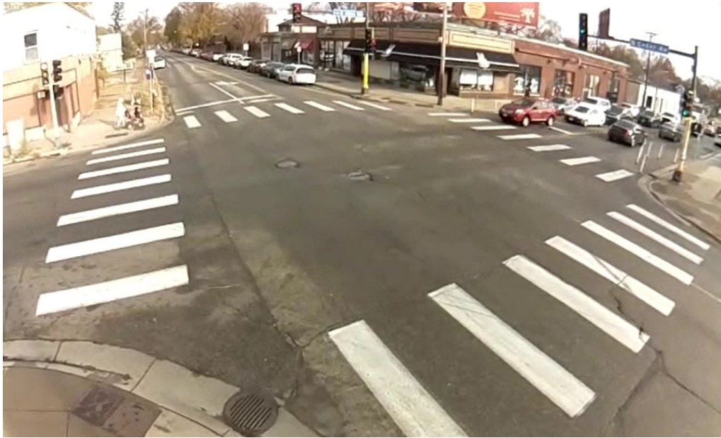
Images of Cedar & 38 th , pre-installation (top image) and post-installation (bottom image).
