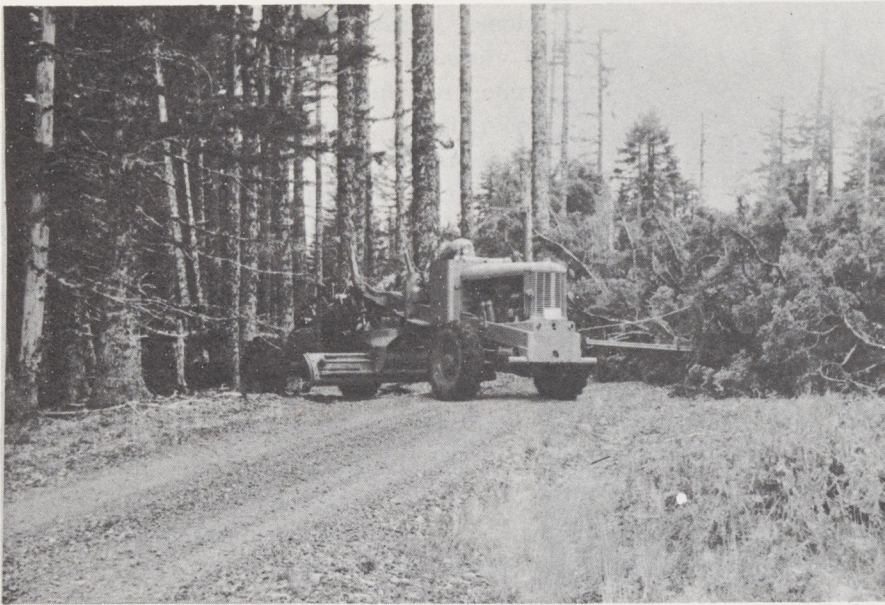
FAA grader (Al Stevens operating) cutting road to by-pass down-falls.
