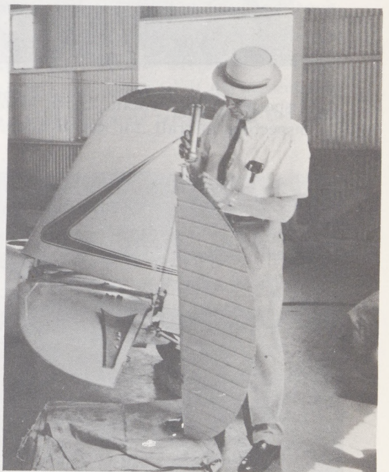
Inspector Harold Buck, Santa Monica, examining defect in elevator as result of improper repair.
