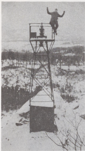
1931. The first side-light of 26 installed in the Columbia River Gorge between Portland and the Dalles, Ore. They were staggered every 3 miles, red on south side of river & green on the north. They were 300 feet above the water and on the cliffs. They were operated by batteries and commercial power.
