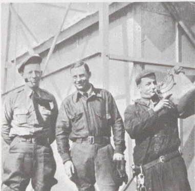
1932. L-R. Cyril T. Hubert, W. G. Edwards & Seth H. Davidson. The first Wind-Aero-Electric installation, and the only one, in the 16th-17th Districts. This site obtained its power from a nine foot propeller driven by the high winds. The generator charged large banks of Edison batteries and the lamps were 32 volts.
