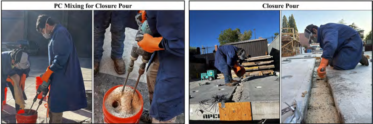
Figure 2.13. PC mixing and closure pour.
