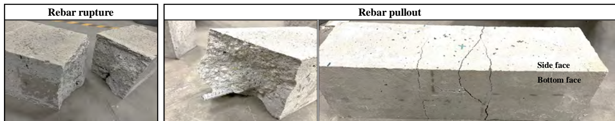
Figure 4.6. Failure mode of beam specimens
