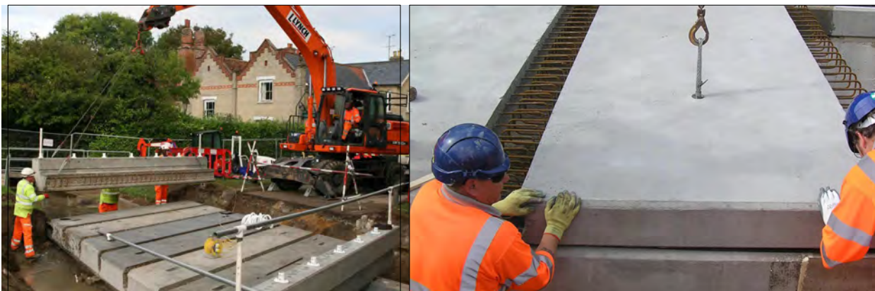
Figure 1.2. Slab girder bridge construction in the United Kingdom [5]
