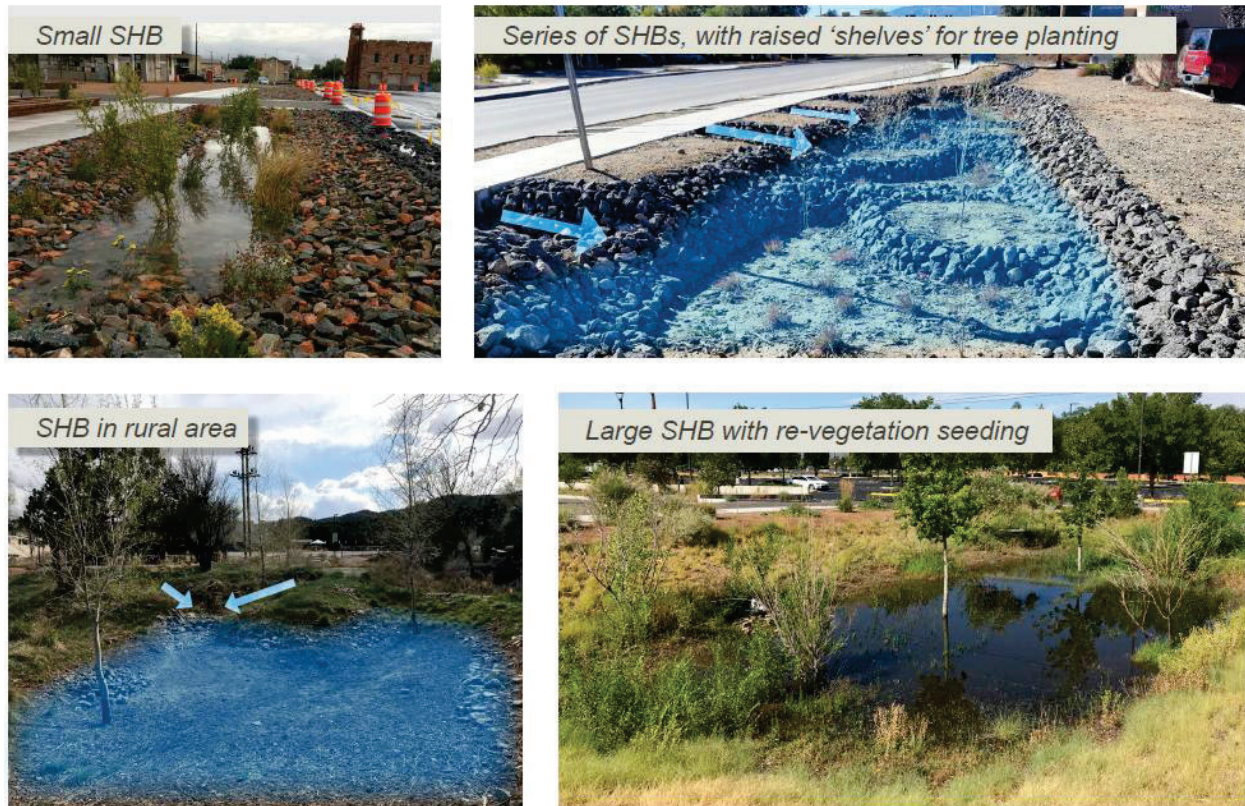
Figure 2 – Stormwater Harvesting Basins, and example of a GI feature from the NMDOT GSI Maintenance Field Guide, (NMDOT, 2024).
