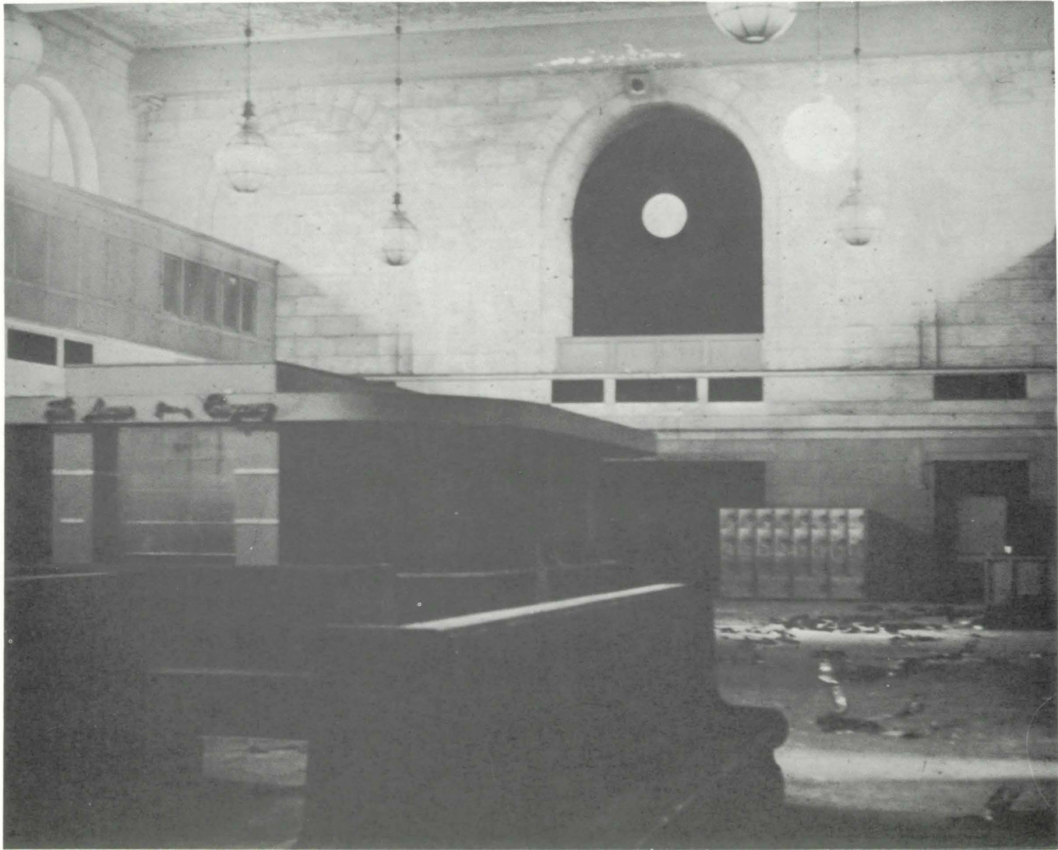
HISTORIC PRESERVATION: Abandoned New Haven Amtrak Station
