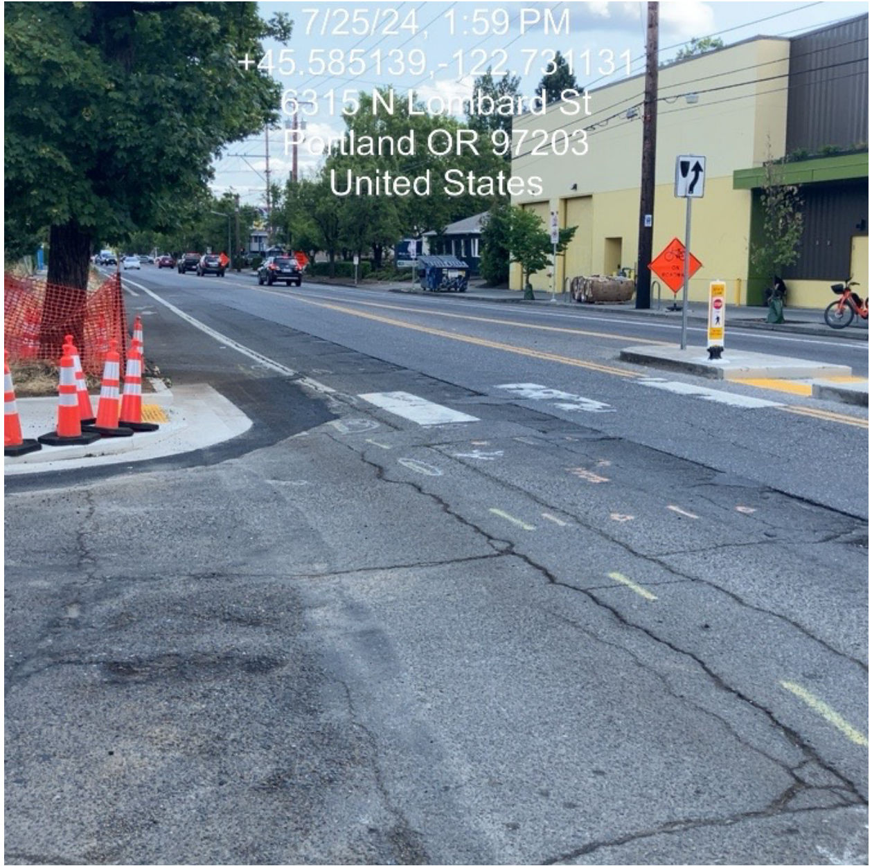
Figure 7.22 N Lombard St and N Fortune St, Portland Stage 2 (R1-6a)
