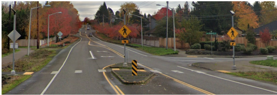
Figure 2.5: RRFB at Rock Creek Trail Crossing on NW West Union Rd.
