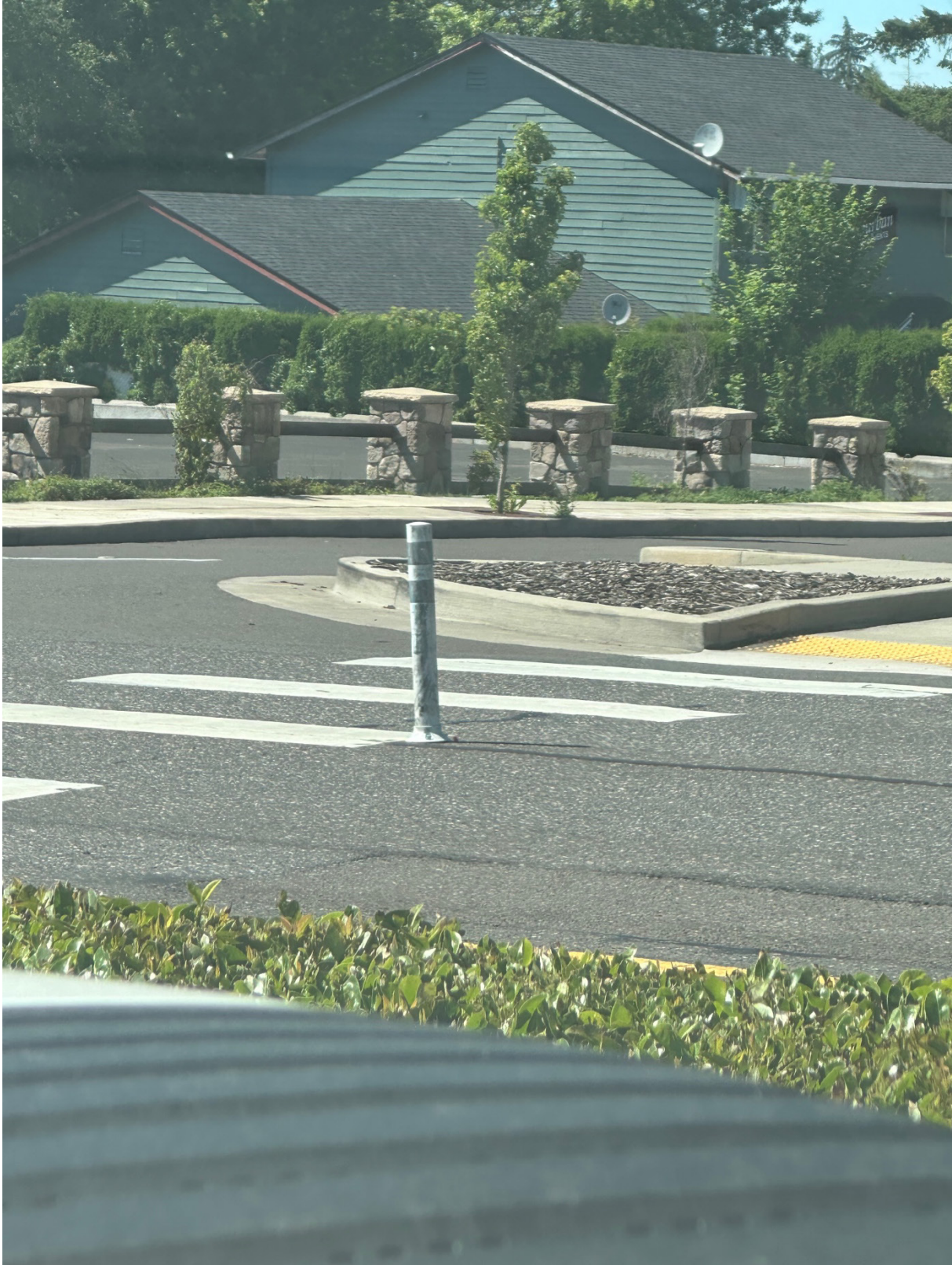
Figure 7.26 Proctor Blvd. and Beers Ave, Sandy Stage 2 (Post on CL)
