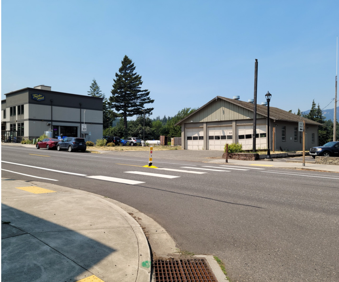
Figure 7.12 Wa Na Pa St. and Regulator St., Cascade Locks Stage 3 (R1-6a)
