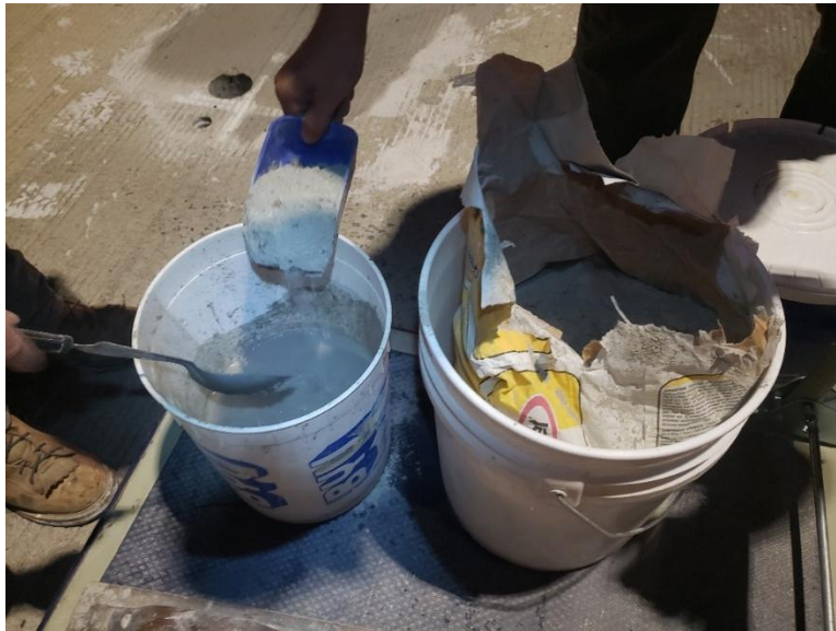
Figure 3.10 Concrete patching.
