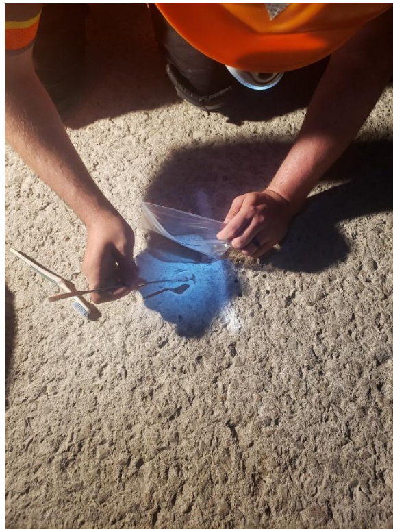
Figure 3.8 Concrete powder sampling.
