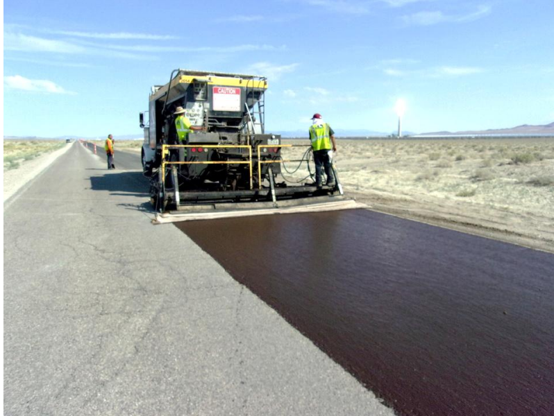
Figure 4. Photo. Application of microsurfacing (Cleaver, 2016).
