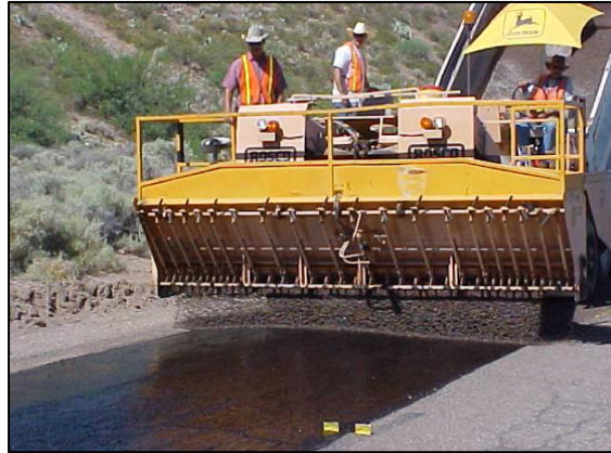
b) Spreading of Aggregate
