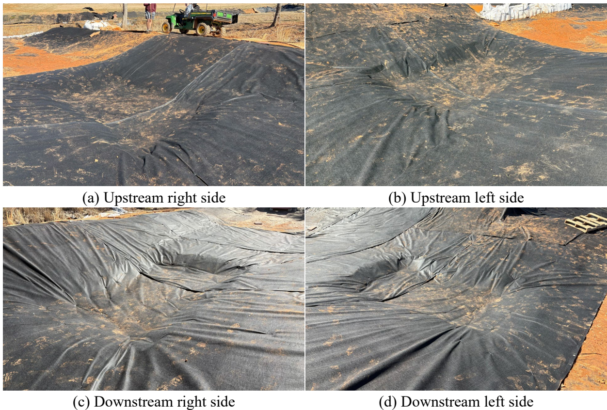
Figure 4.1: NDOT Standard Silt Trap
