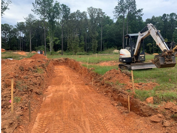
(a) Excavating Stage
