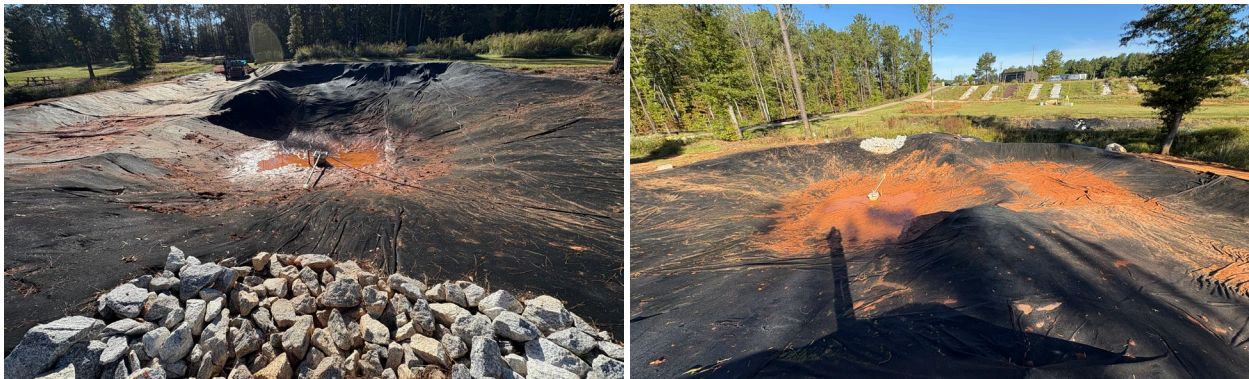
(a) Sediment Trap from Weir
