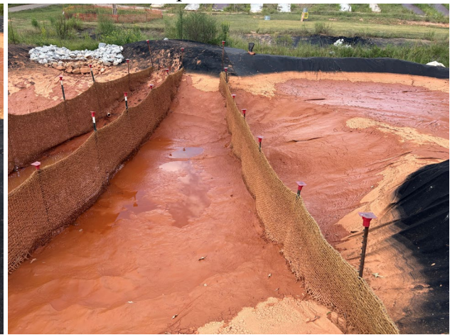
(c) Second Bay of Sediment Trap
