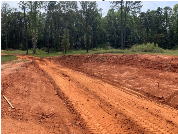
(c) Fine Grading Stage
