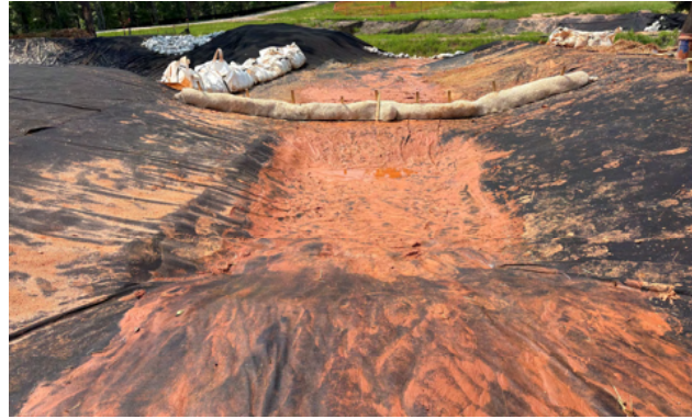
Note: pictured on upstream side facing downstream in channel
