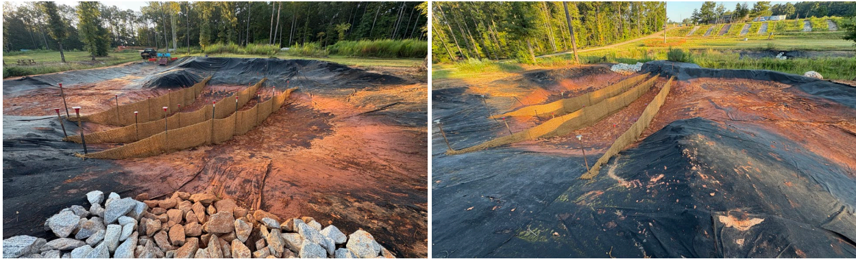
(a) Sediment Trap from Weir
