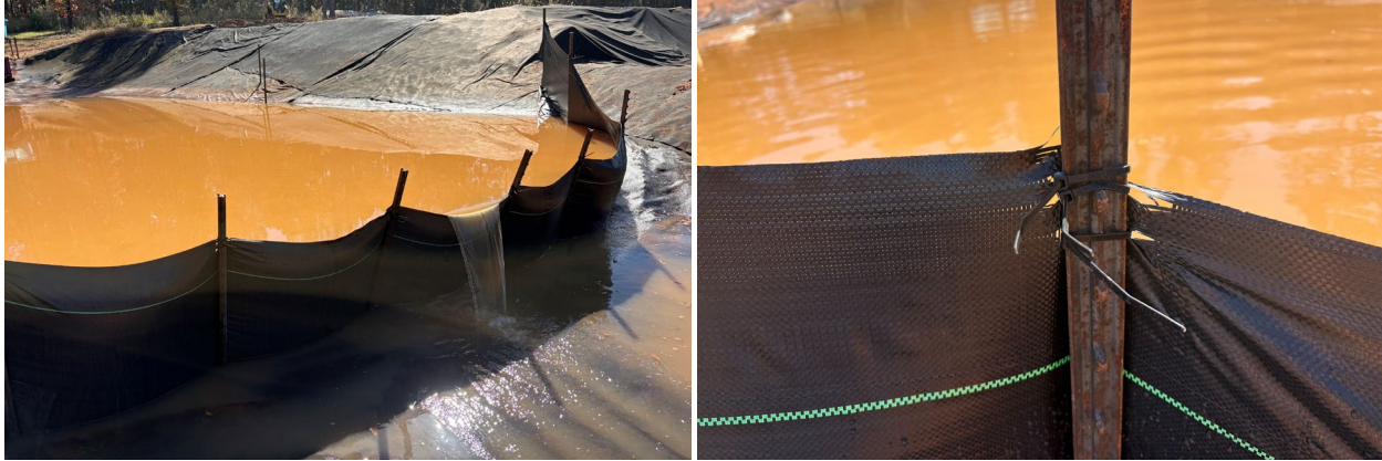
(a) Installation behavior
