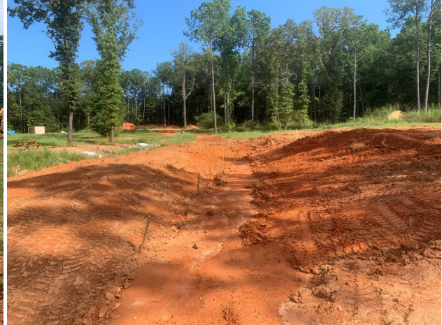
(b) Rough Grading Stage
