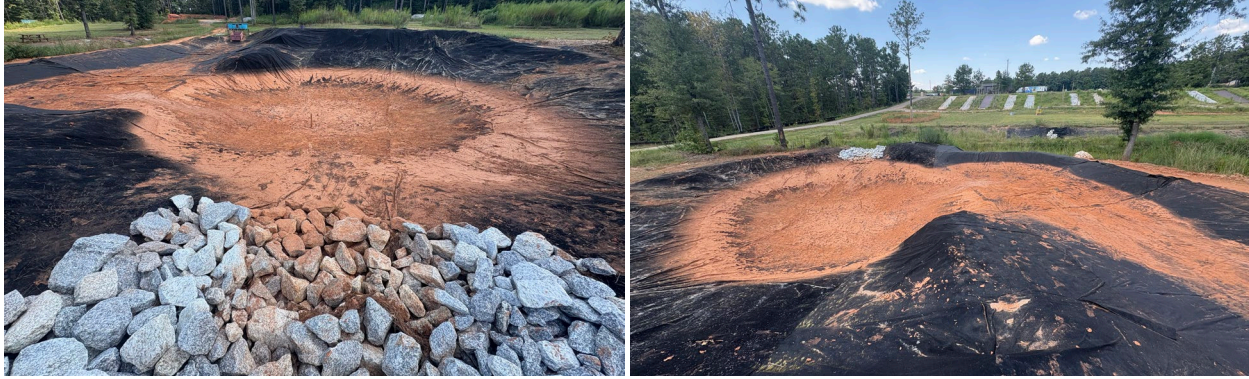
(a) Sediment Trap from Weir
