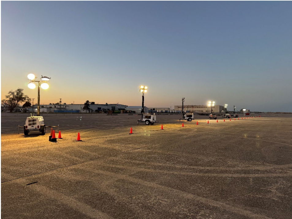
Figure 3.8 Light Tower on Site Set Up
