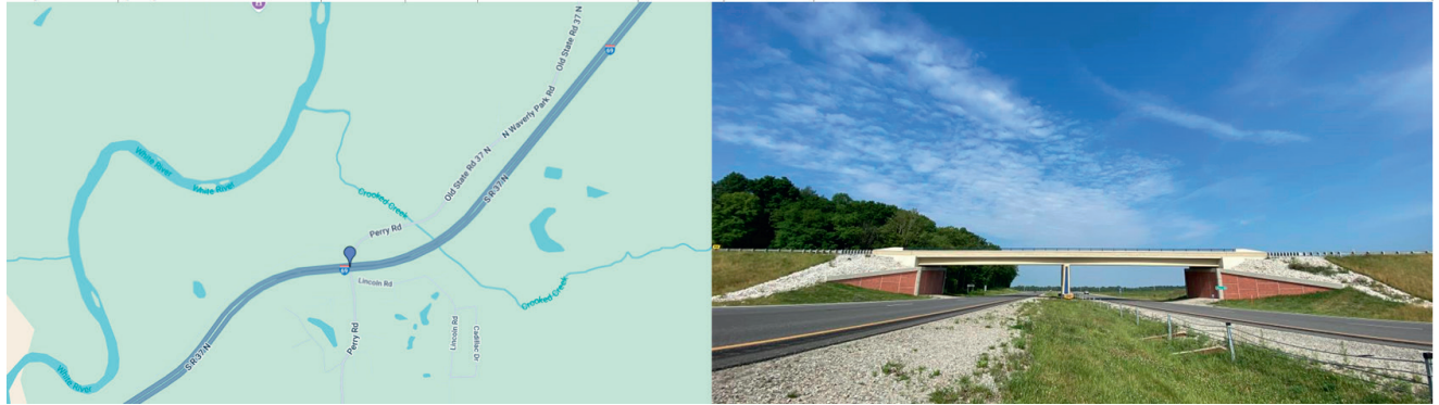
Figure 4.14 Low-Score Bridge: Asset (37)I69-55-10531 (iTAMS, 2025; Maps Data: Google ©2025).
