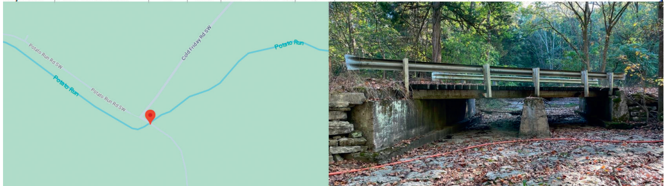
Figure 4.15 Low-Score Bridge: Asset P000-31-07079 A (iTAMS, 2025; Maps Data: Google ©2025).
