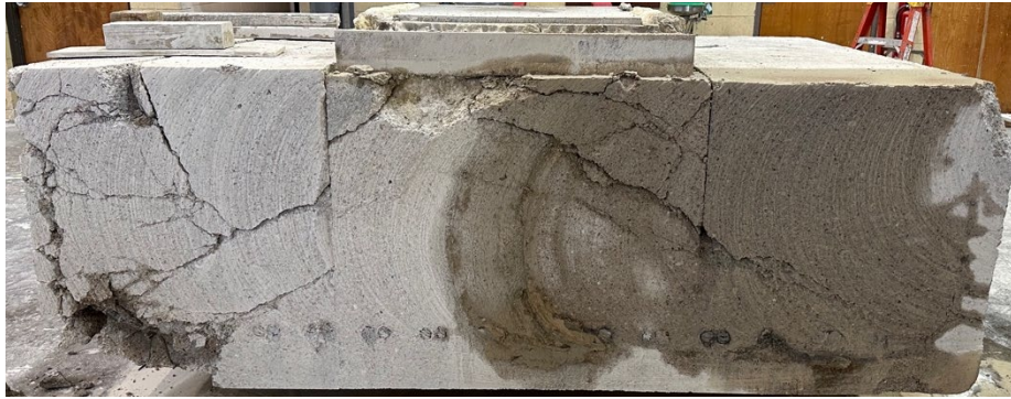
(a) Crack patterns at the cold joints after sectional cut
