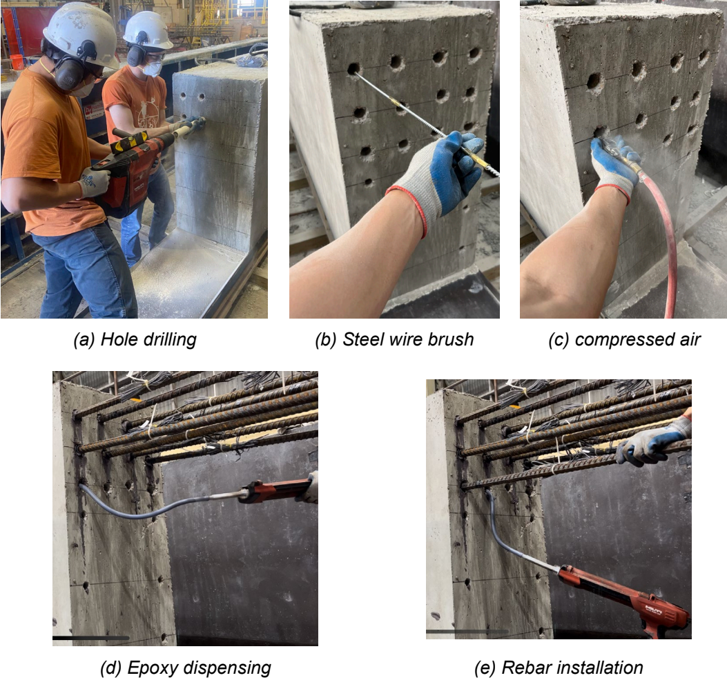
Figure 5-17 Installation procedure for dowel bars
