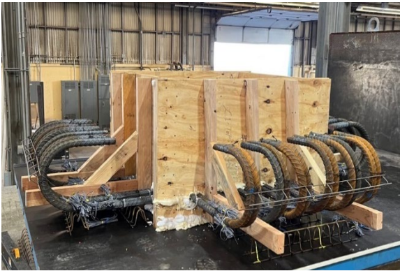
(a) Steel cage and wooden formwork fabricated for the internal section
