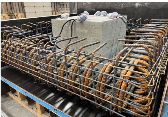
(c) Steel cage fabricated for the external section
