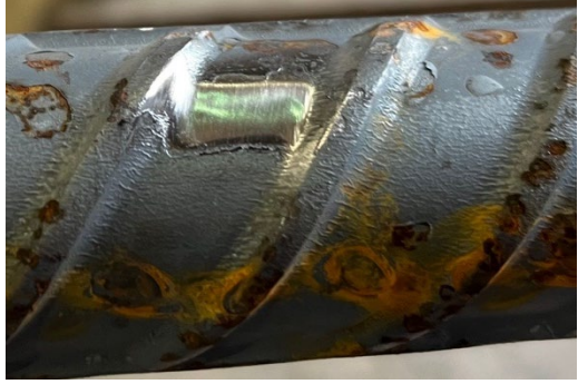
(a) Rebar surface after grinding
