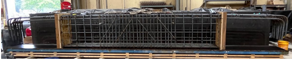
(a) Steel cage fabricated for the interior section
