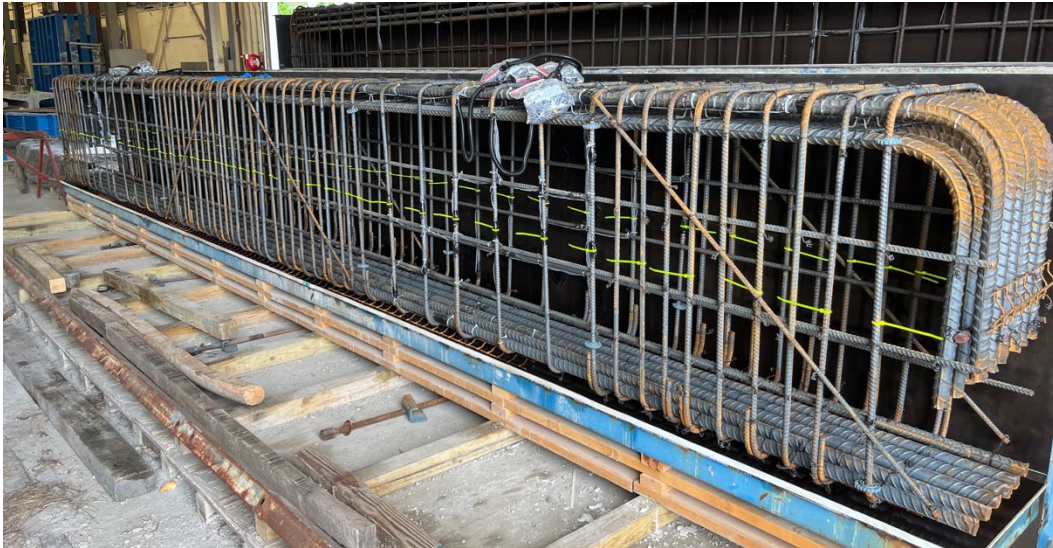
Figure 5-14 Steel cage of I-1.85-03-H and I-1.4-03-H
