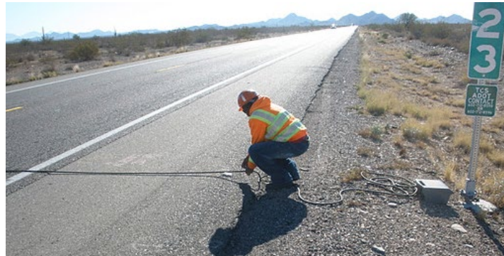
Figure 1. Pneumatic Traffic-Counting Device Installation
