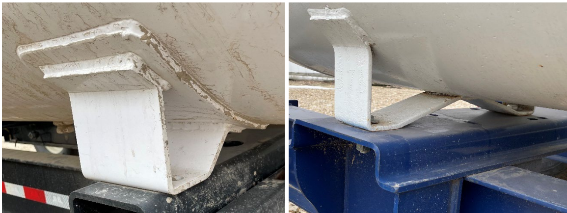
Figure 10. Face-to-tank Foot attached via Pad (left) and Directly to Tank (right)
