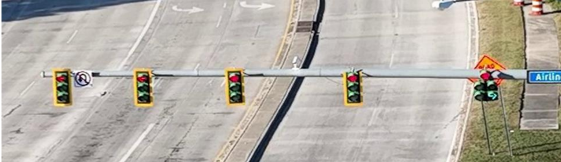
Figure 16. Traffic light at Plank Road at 72nd Avenue; from left: Y/G-Protected and R/Y/G
