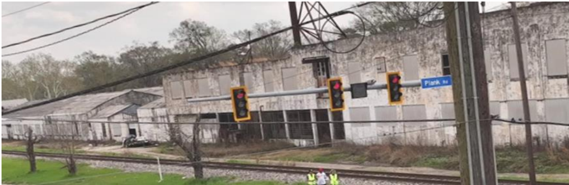
Figure 18. Traffic light at Plank Road at Choctaw Drive: All R/Y/G
