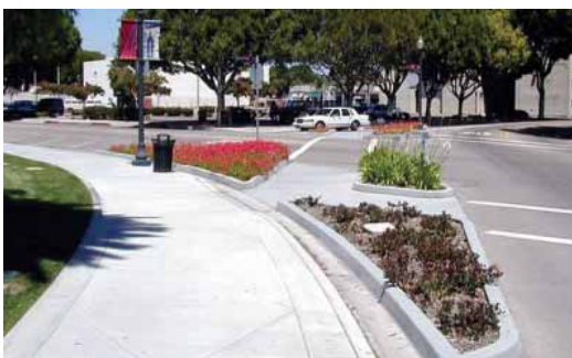
Wide radii (top) allow faster turning speeds and create unsafe pedestrian environments. A simple extension (bottom) can reduce the turning radius and vehicle turning speed as well as provide a safer crossing place for pedestrians.
