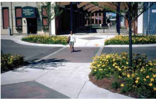
Curb extensions can increase the visibility of pedestrians and motorists.
