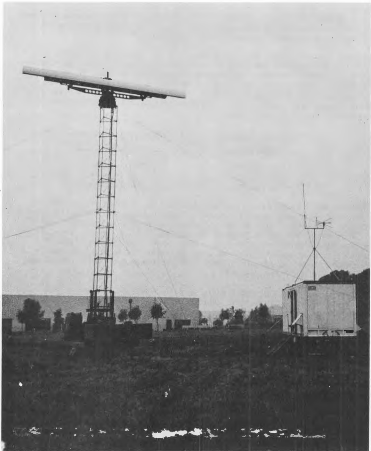
FIGURE 5. SITING SYSTEM ANTENNA TOWER AT 48FT. +1/2'
