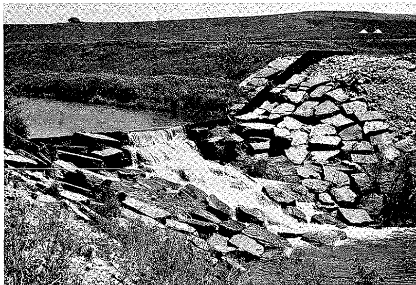
Plate 8. Grade stabilization structure consisting of a single row of sheetpile reinforced with derrick stone.
