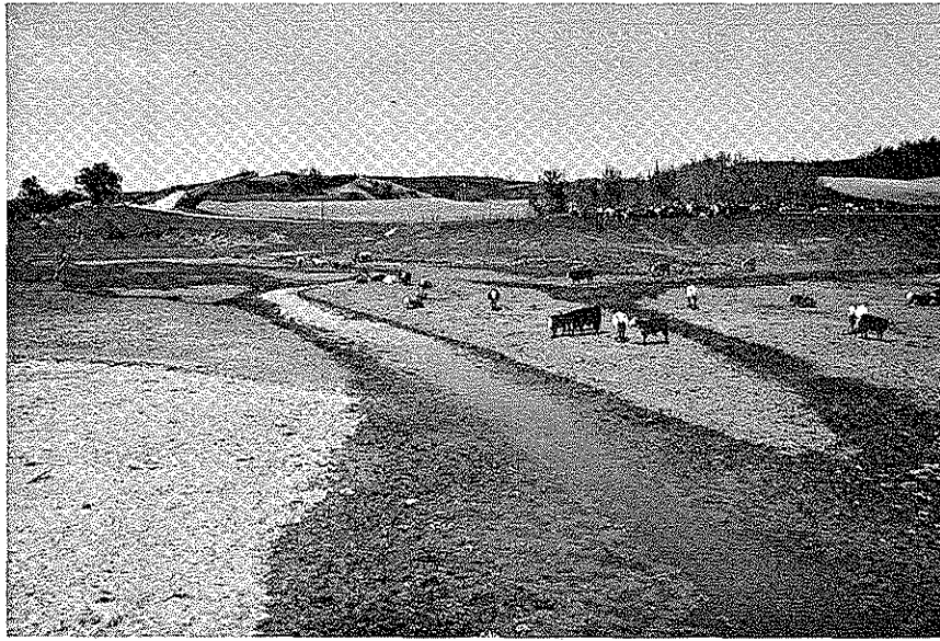
Plate 15a. The aggraded prism of sediment deposited upstream of a flume bridge in Monona County. Compare this photo with the downstream view in 15b.
