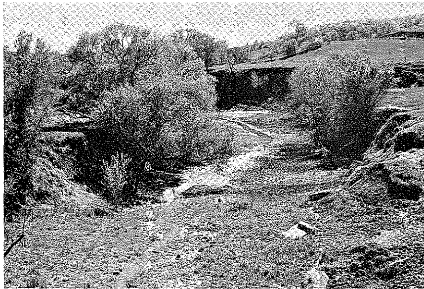
Plate 15b. A degraded channel downstream from a flume bridge. Compare this photo with the upstream view in 15a.
