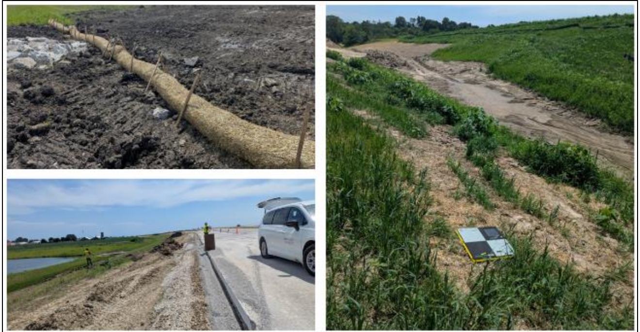
Figure 5. Erosion and sediment control devices at Mediapolis Site 2, including wattles, a reseeded slope, and a check dam
