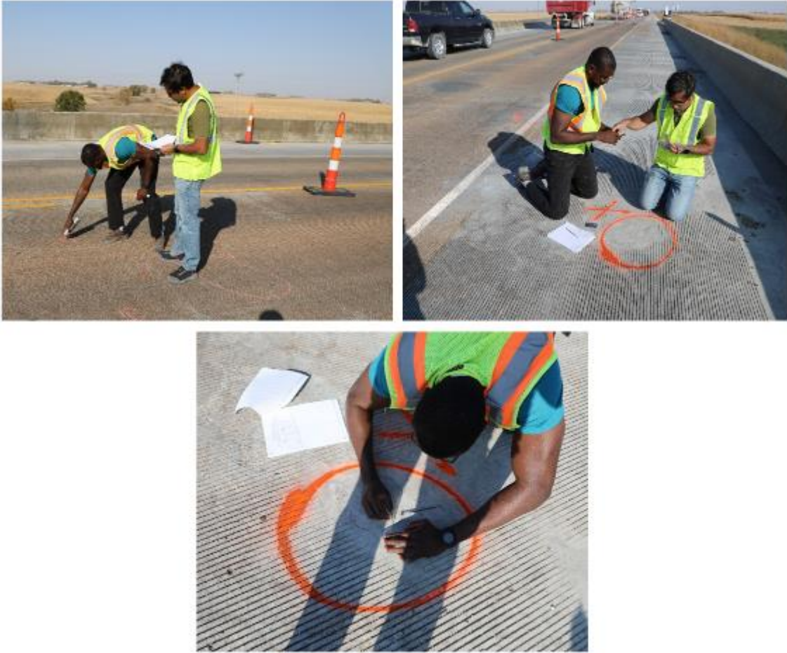
Figure 43. Research team manually inspecting the bridge and marking identified cracks
