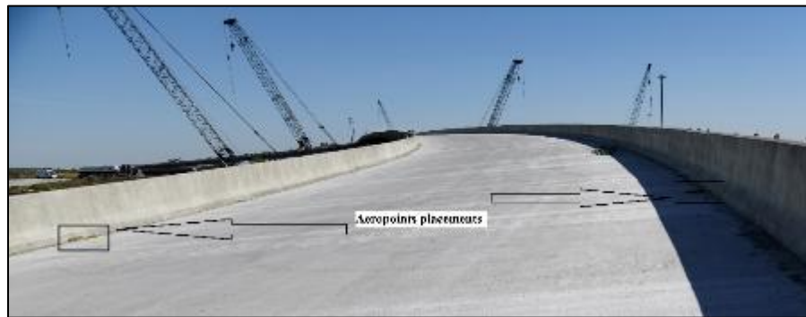
Figure 8. Placement of AeroPoints GCPs on the ground
