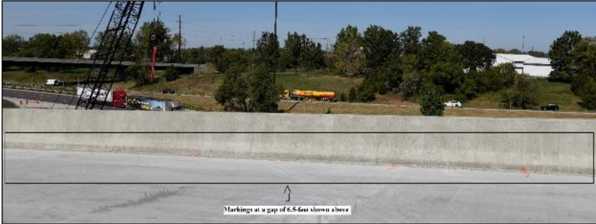
Figure 9. Markings at intervals of about 6.5 ft for an appropriate overlap
