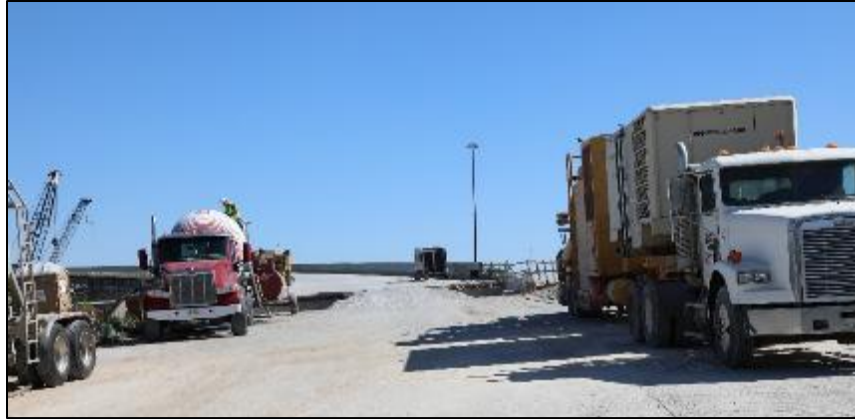
Figure 6. Presence of heavy construction equipment
