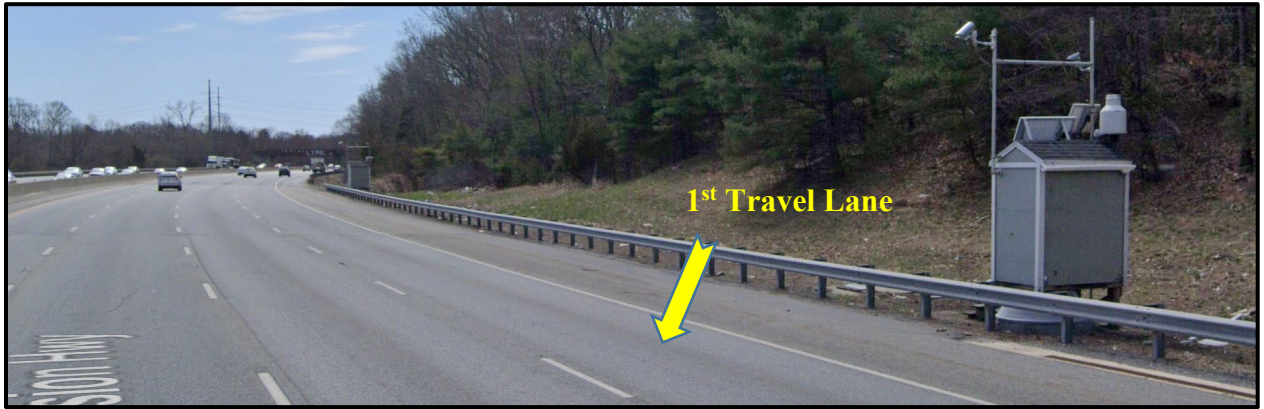
Figure 2.8: Lane for installation of invasive sensors
