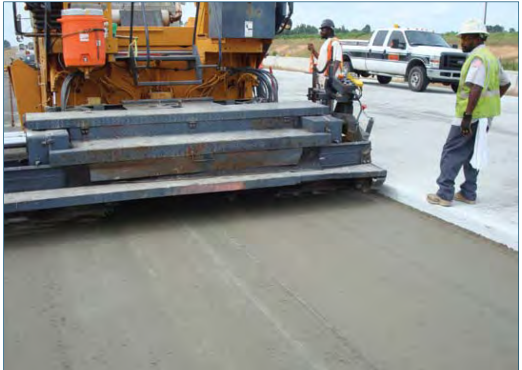
Figure 7-4. Close-up view of paver
