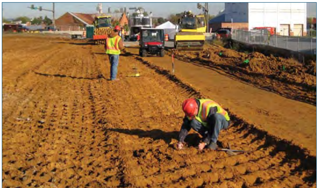
Figure 7-1. Preparation of subgrade
