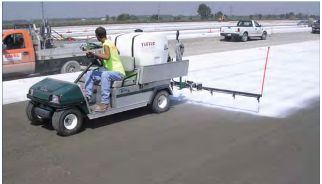
Figure 7-16. Application of curing compound
