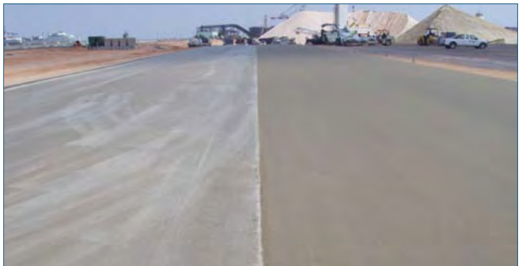
Figure 7-14. Longitudinal construction joint
