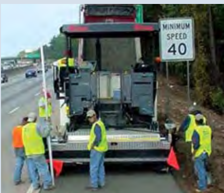
Interstate highway shoulder, Atlanta, GA
