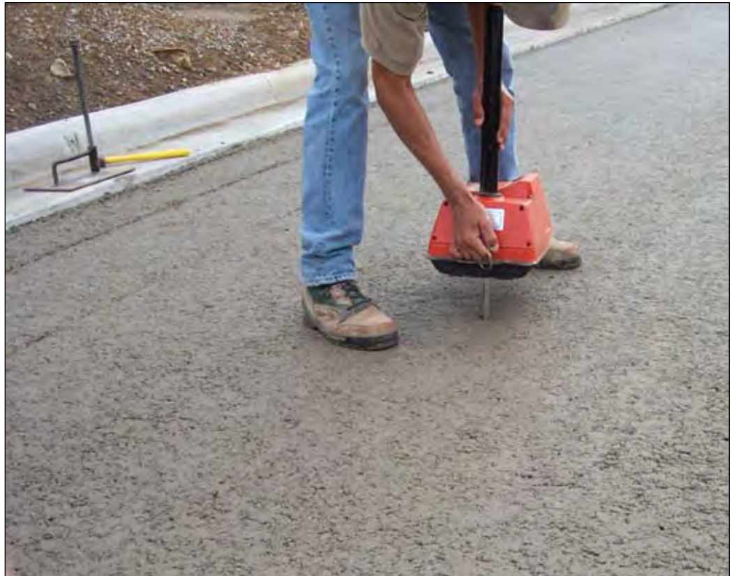
Figure 7-3. Checking density using a single-probe nuclear gauge
