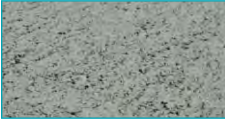
Mix too dry
