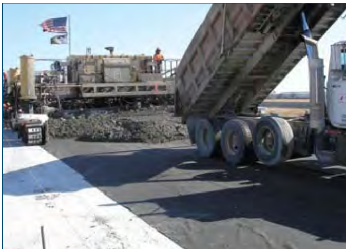
Figure 2-7. Concrete paving with geotextile fabric layer
