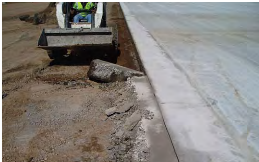
Figure 7-7. Finished longitudinal construction cold joint
