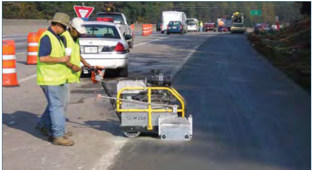
Figure 7-13. Shoulder transverse sawed joint
