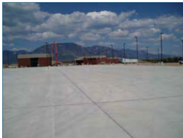
Figure 7-12. Sawn transverse and longitudinal joints
