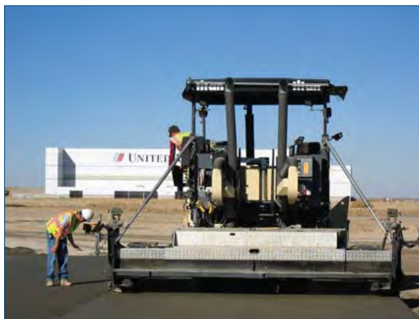
Figure 2-3. RCC paving operation at an airport
