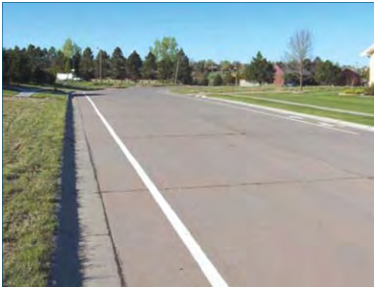
Figure 2-5. RCC pavement used for a local street
