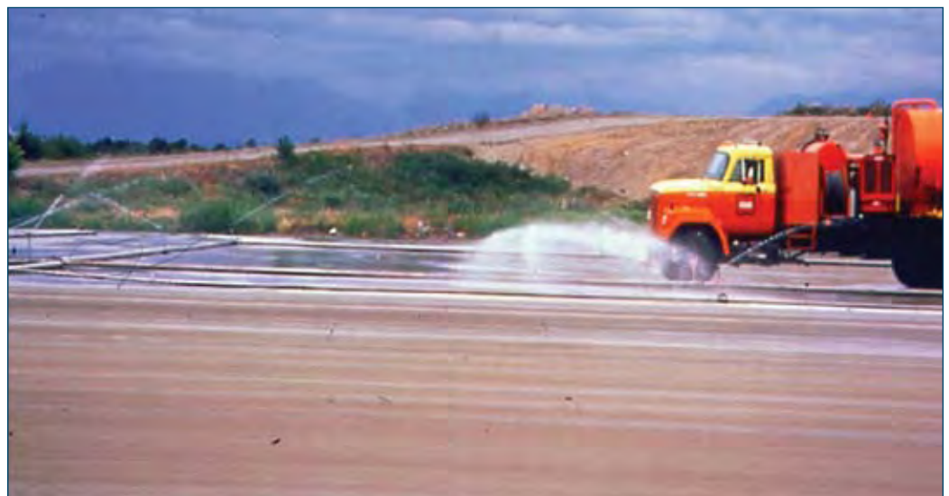
Figure 7-17. Moisture curing using sprinklers and fog spraying
