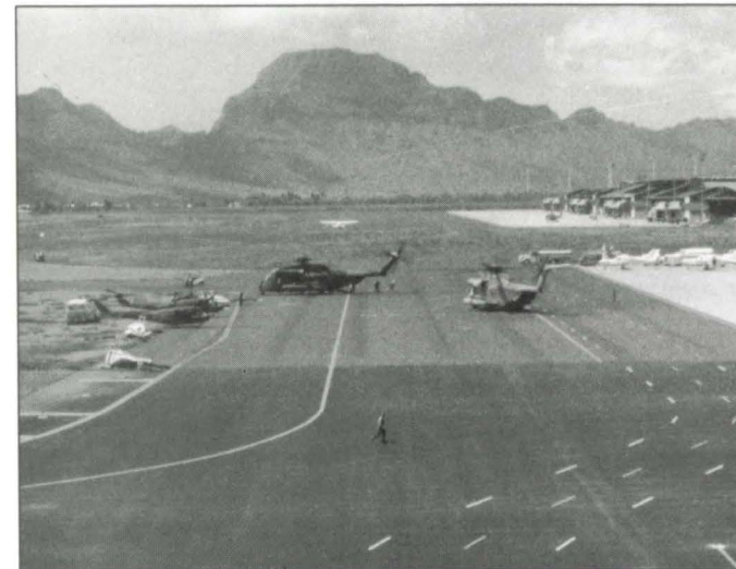
Lihue Airport was in the path of Iniki.
