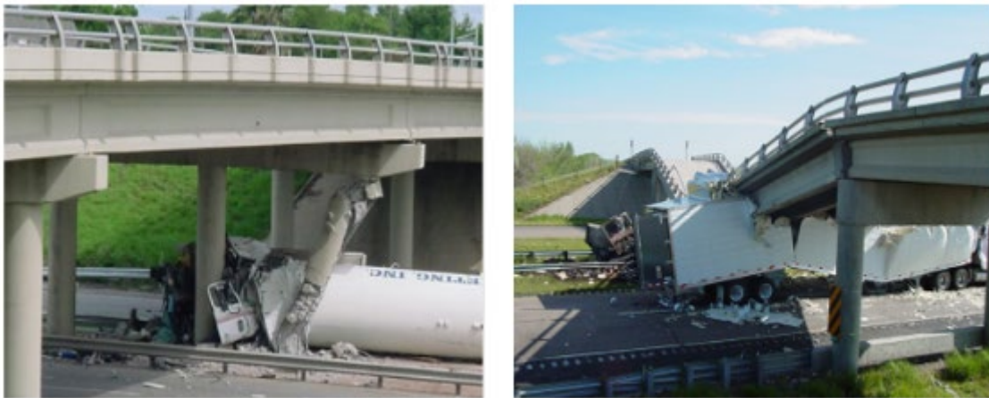
Figure 1.1: Failure of Bridge Structures Due to Vehicle Collisions
