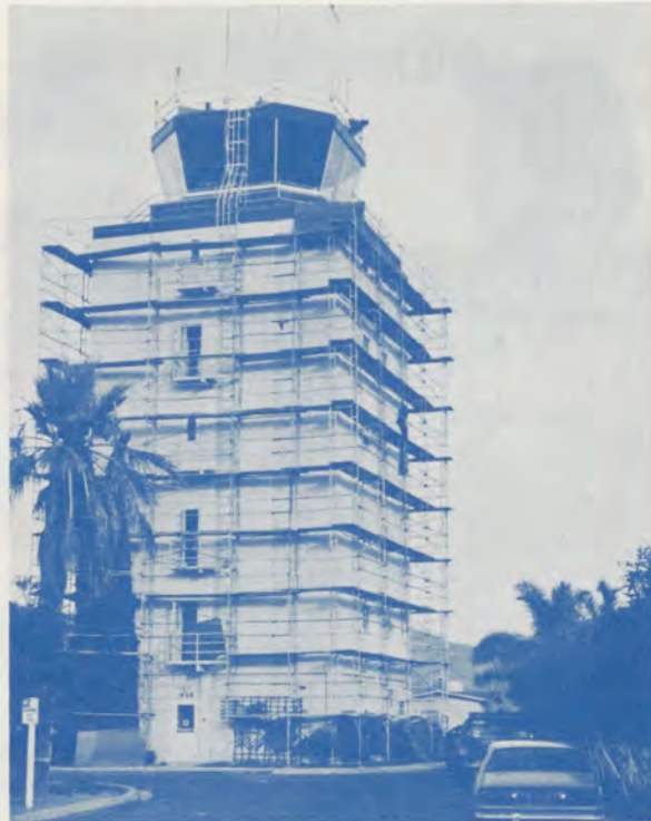
Gillespie Tower during application of exterior treatment.
